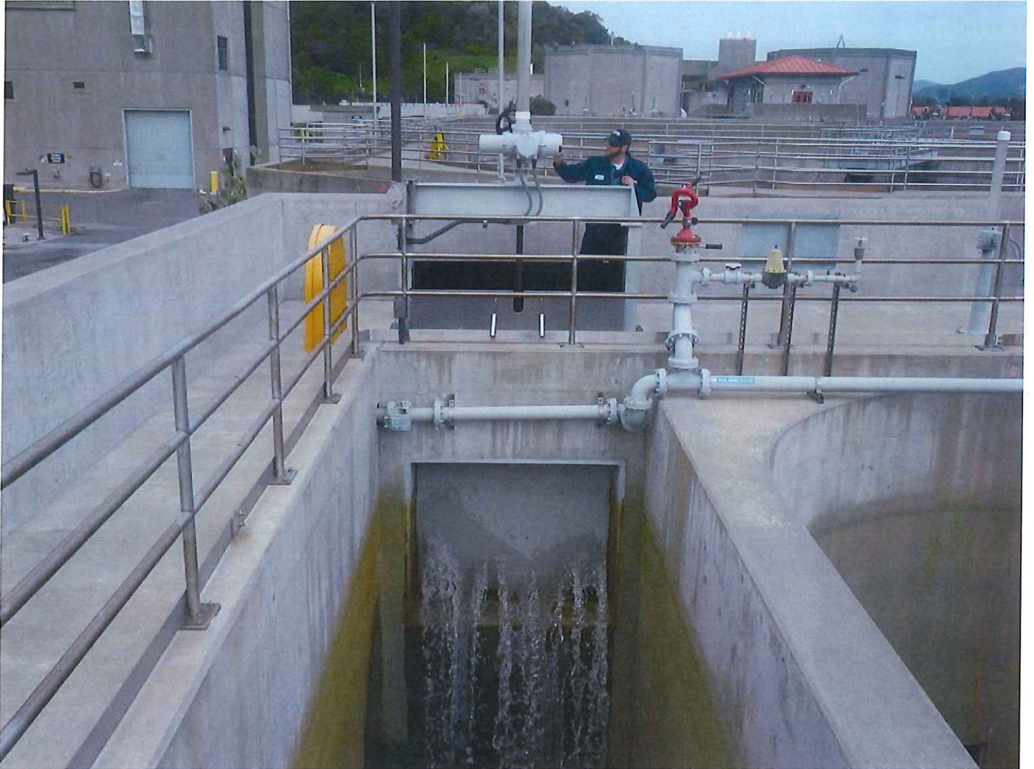
Operator Jeremy Schwarm preparing contact tanks for wet weather use.
