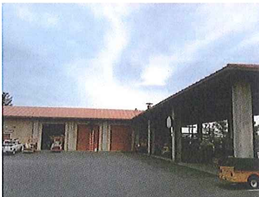
Maintenance Building and Covered Portico
