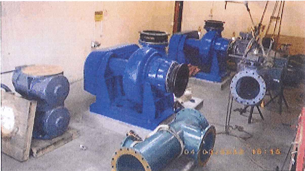
DIGESTER IMPROVEMENT PROJECT NEW MIXING PUMPS
