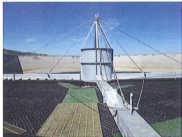
New rotary distributor, Biotower No. 2
