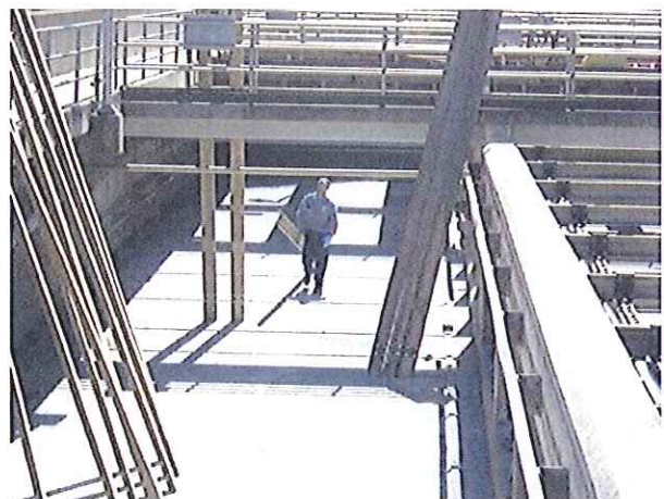
Primary Clarifier No. 1 being retrofitted.
