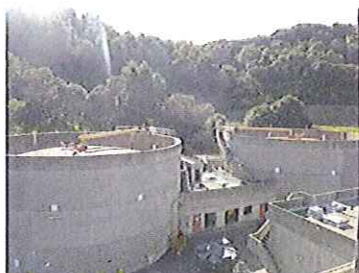
Digesters, showing existing floating steel covers
