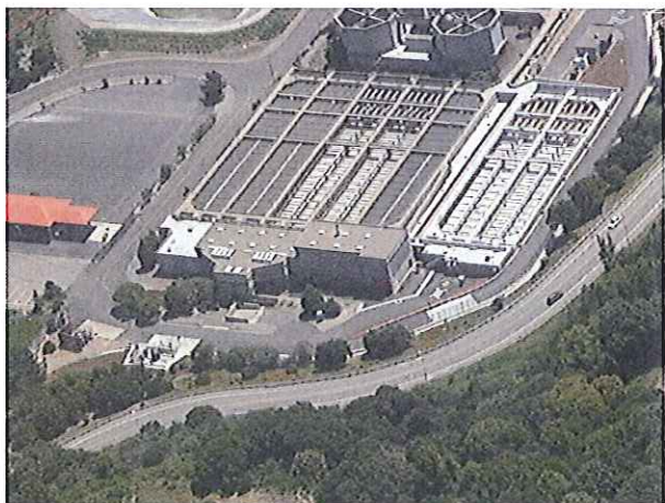
Aerial View of Primary Clarifiers
