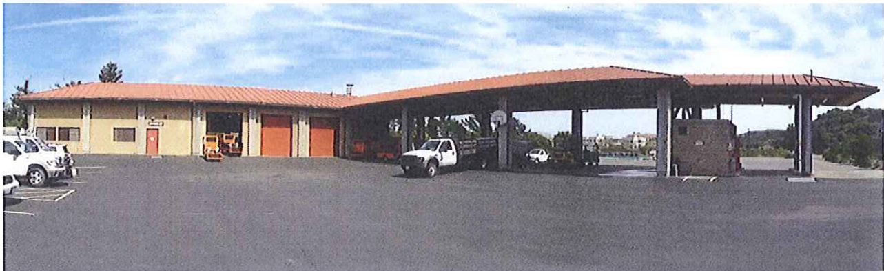
Maintenance Building with Standing seam metal roofs.
