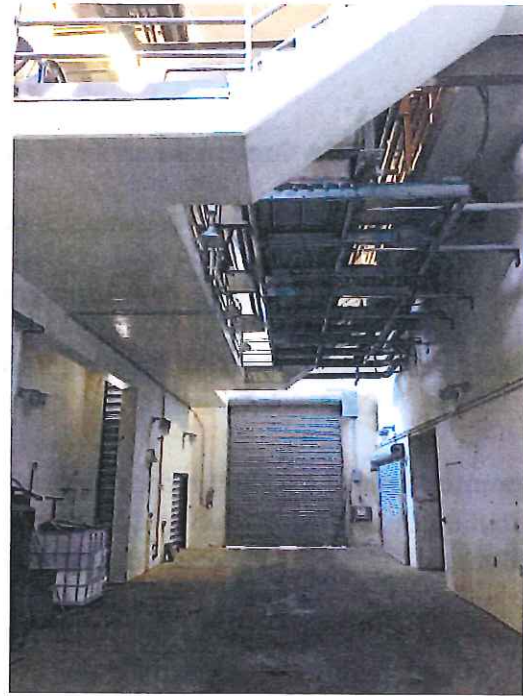
Biosolids truck loading area and hoppers
