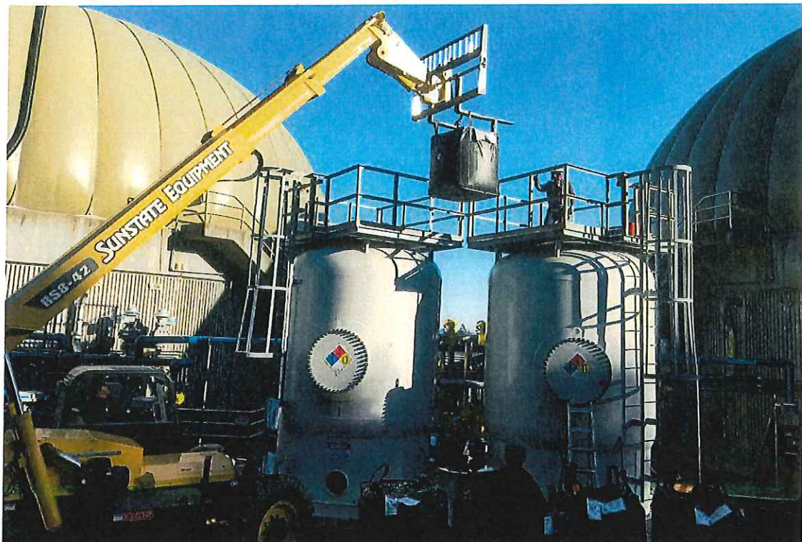
Biogas conditioning media replacement
