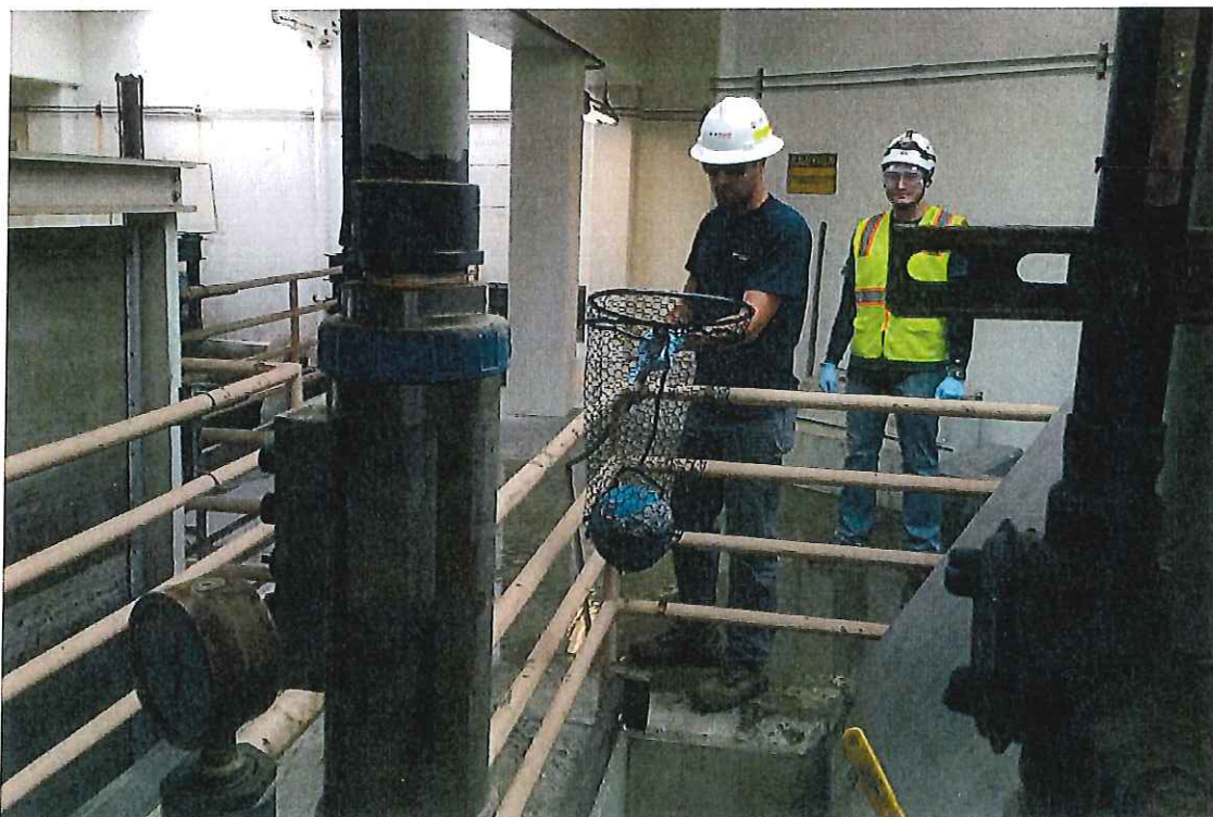
Ross Valley Interceptor assessment "Smart ball" extraction from Agency headworks
