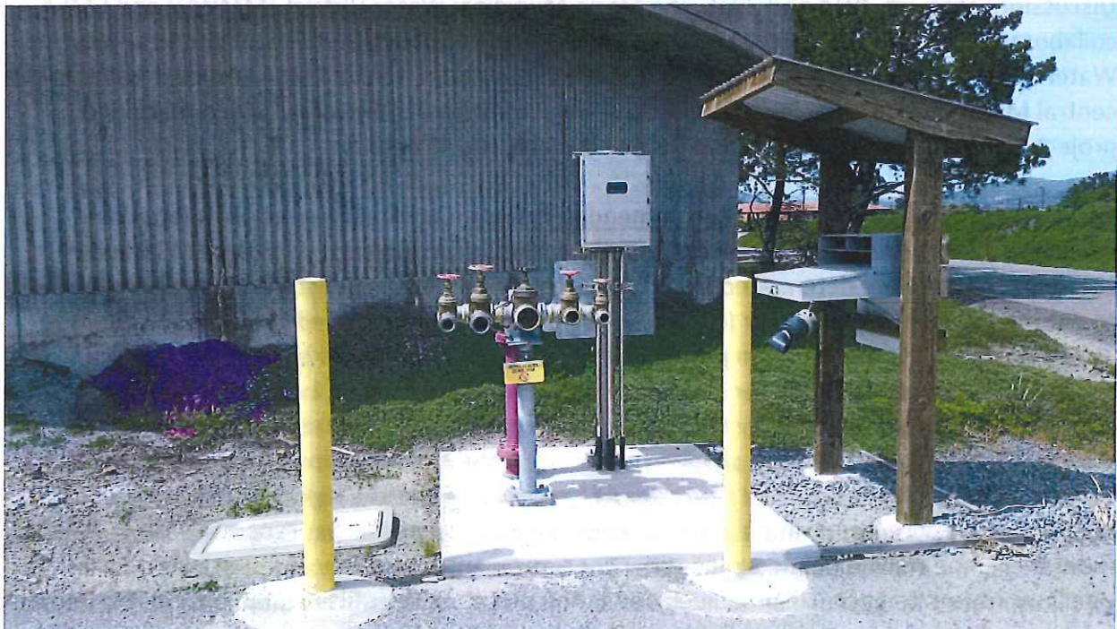
CMSA Recycled Water Truck Filling Station
