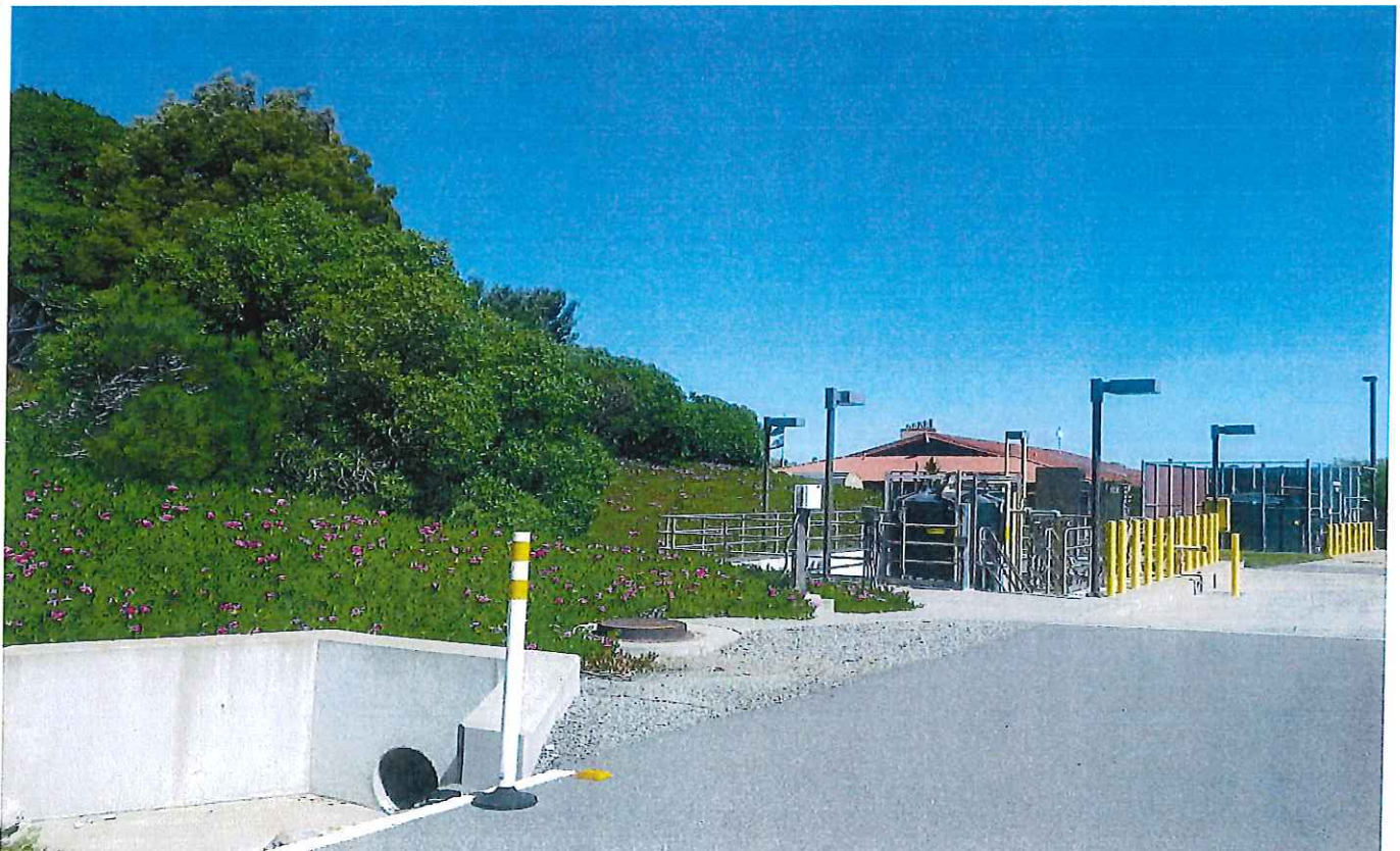
Hillside near the treatment plant headworks
