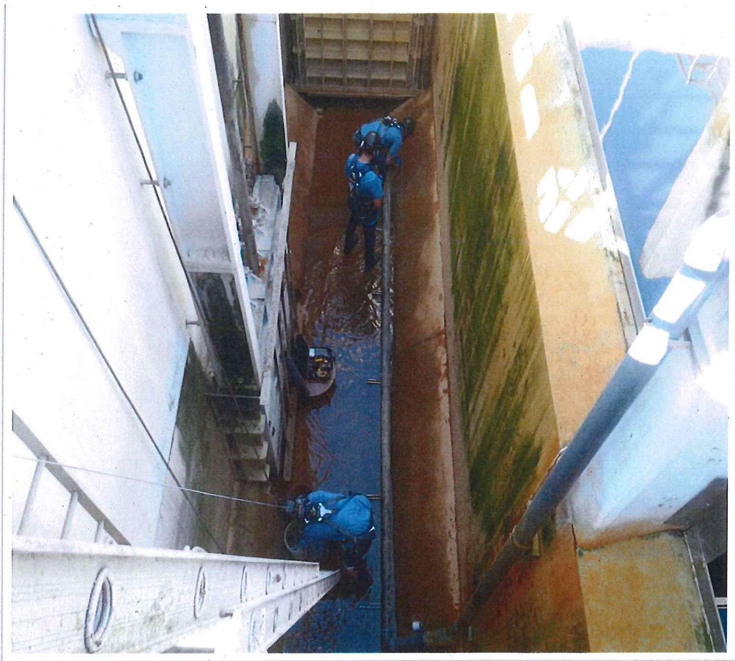
Technicians Performing Annual Maintenance and Repairing a Dechlorination Line in the Outfall Sump
