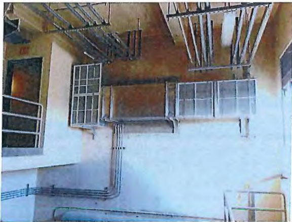
Figure 5 – New supply duct on SHB interior
