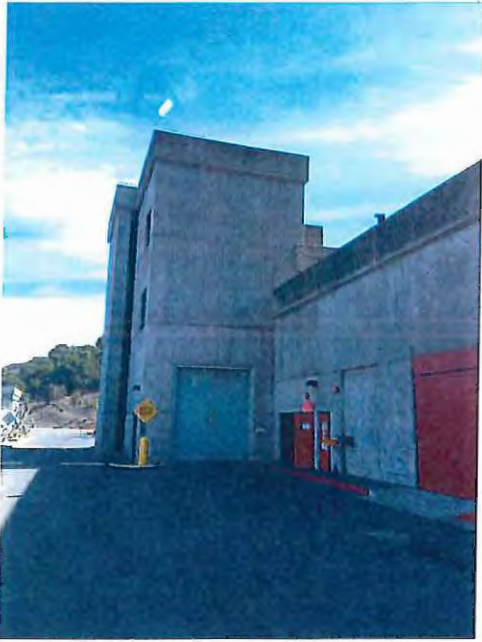
Figure 3 – Original SHB exterior (east view)
