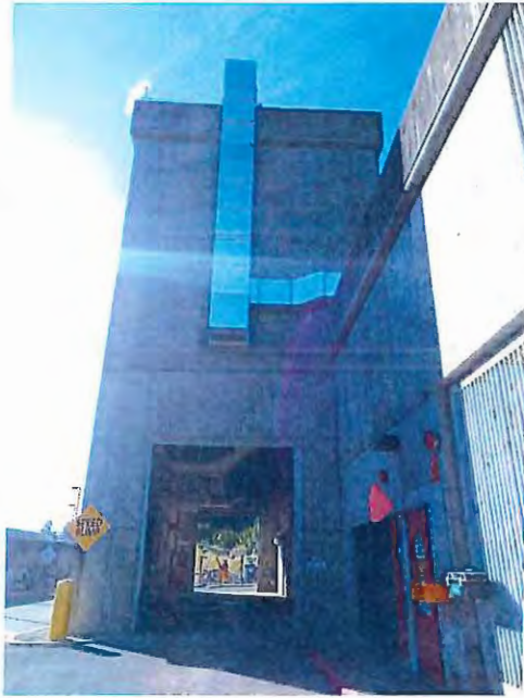
Figure 4 – New supply duct on SHB exterior
