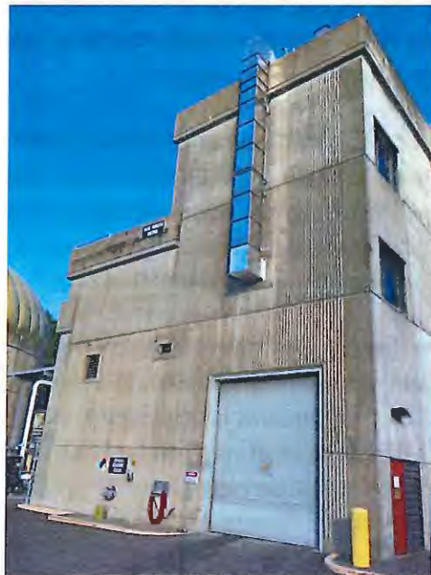
Figure 2 – New exhaust duct on SHB exterior
