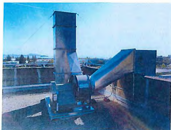
Figure 8 – New exhaust fan on SHB roof
