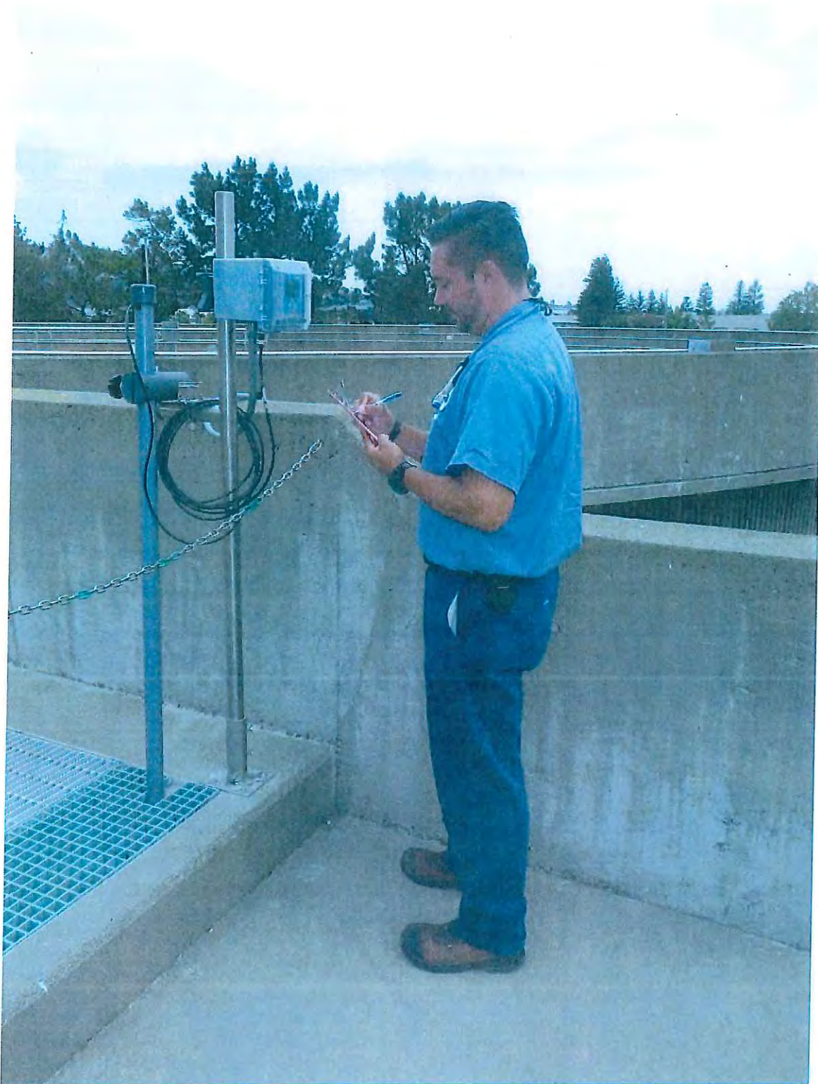
Operator Nick Gaunt Verifies Instrumentation Accuracy during Daily Operational Checks
