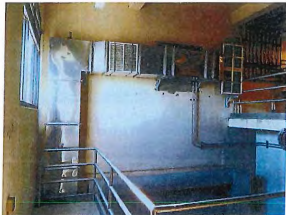
Figure 6 – New exhaust duct on SHB interior
