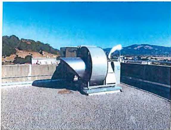
Figure 7 – New supply fan on SHB roof
