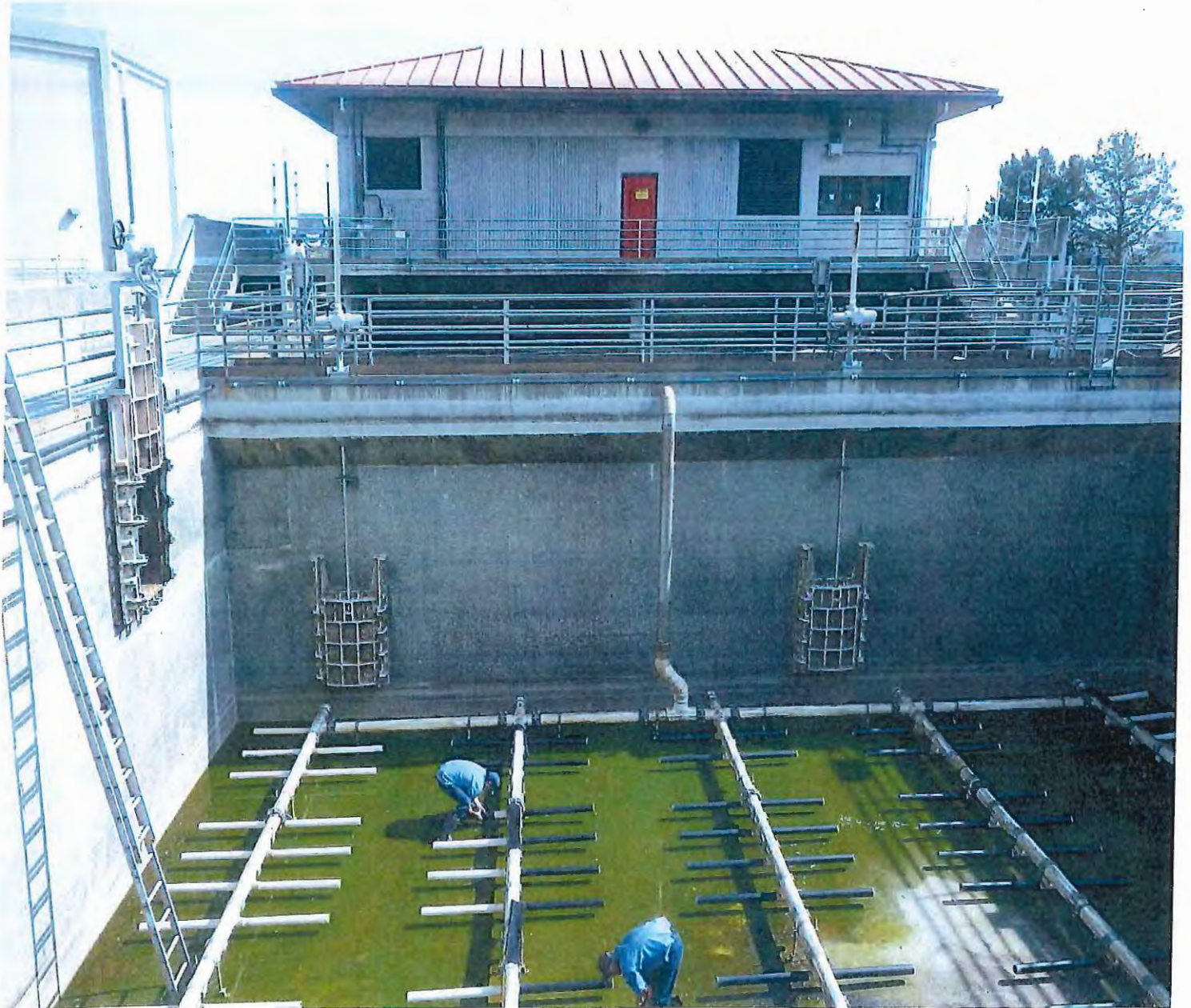
Technicians Replacing Diffuser Membranes in Aeration Basin No. 1
