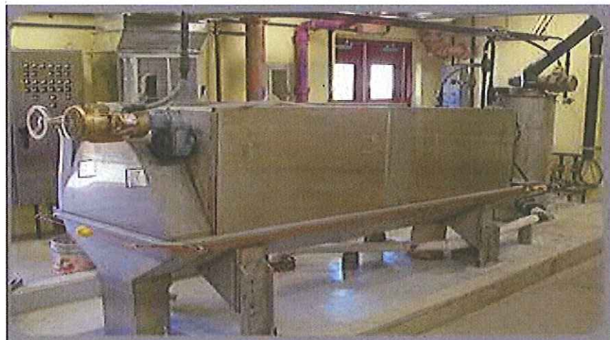
Typical Rotary Drum Thickener Installation
