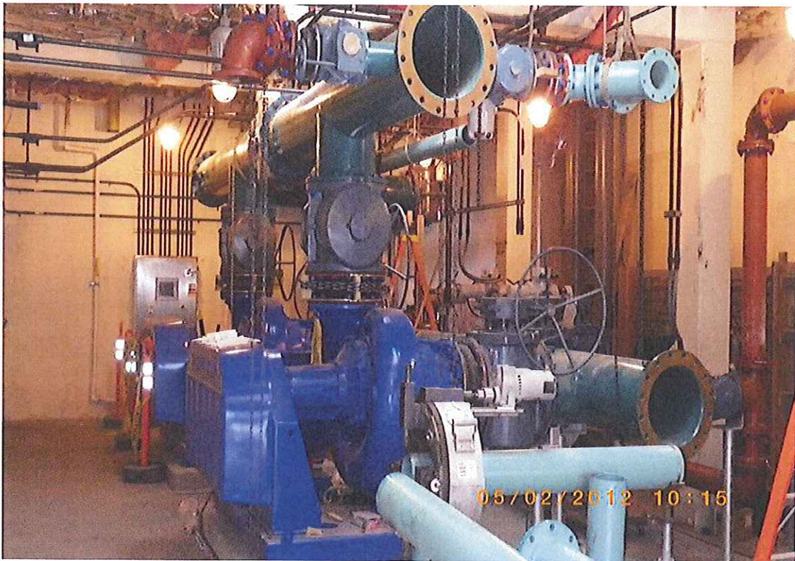
Digester Improvements Project Pumps and Piping Installation
