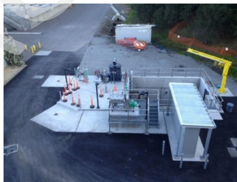
Organic Waste Receiving Facility
