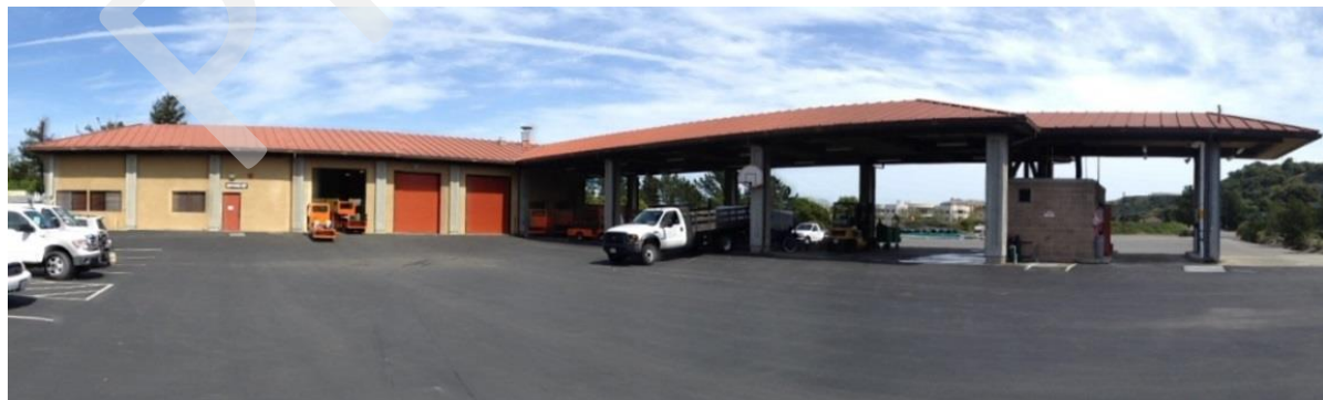
Maintenance Building with standing seam metal roofs.
