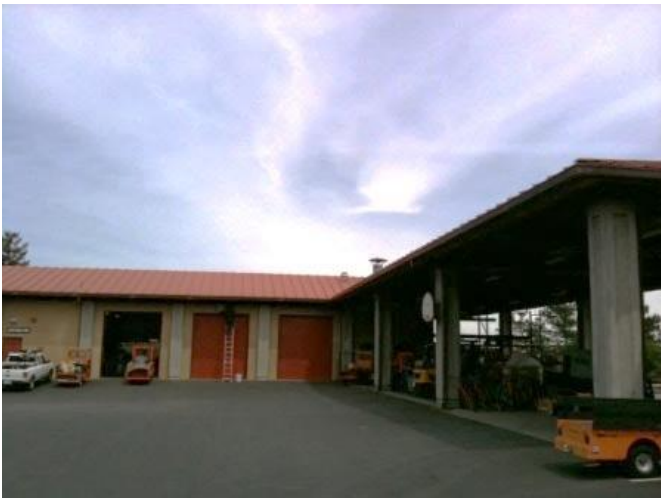
Maintenance Building and Covered Portico
