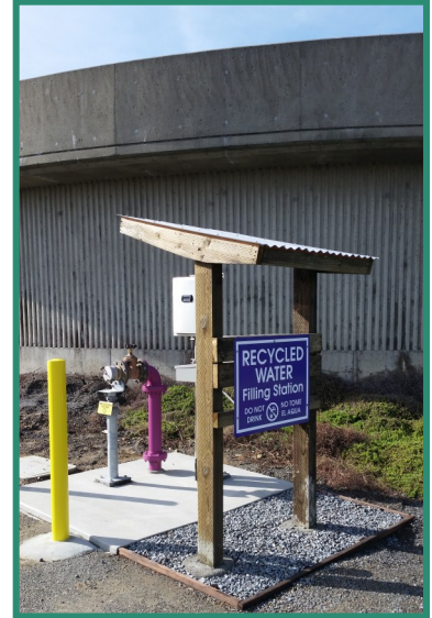
Recycled Water Truck Fill Station.
