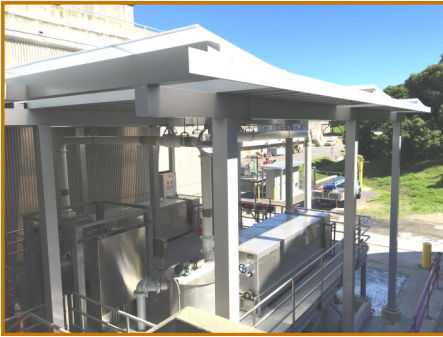
Newly installed RDT's under new canopy.
