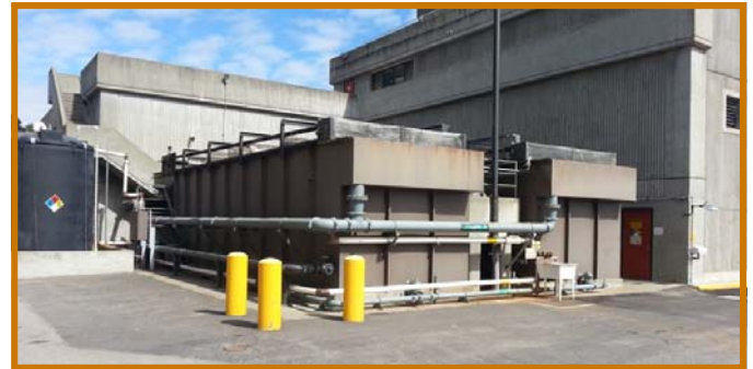
Existing dissolved air flotation thickeners (DAFs) to be replaced.
