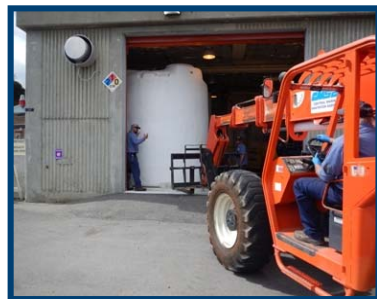
Staff installs the SBS tank with the help of the SkyTrak lifter.
