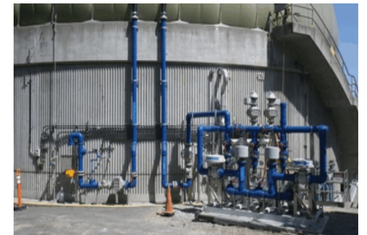
New membrane cover system piping and compressors.
