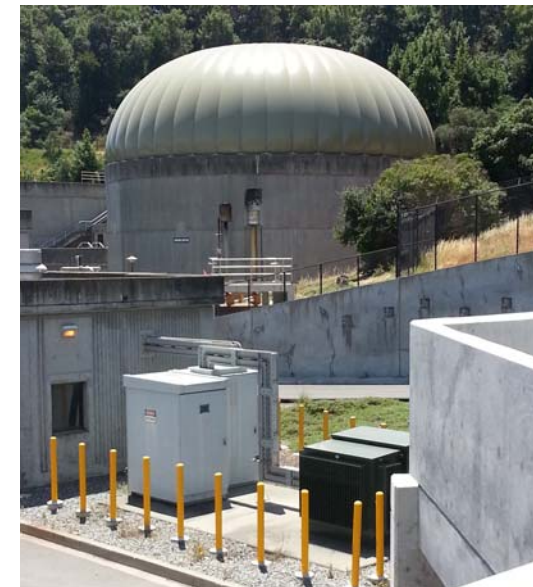
Digester No. 1 with membrane cover.
