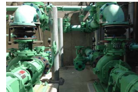
New FOG/Food Waste receiving station pumps.
