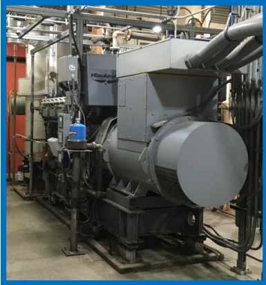
Agency's existing cogeneration engine.
