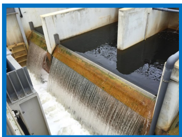
New weirs in service.
