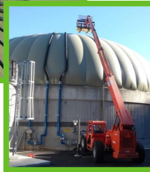
Rough terrain forklift and man-rated basket used to install Laser Level protection system.
