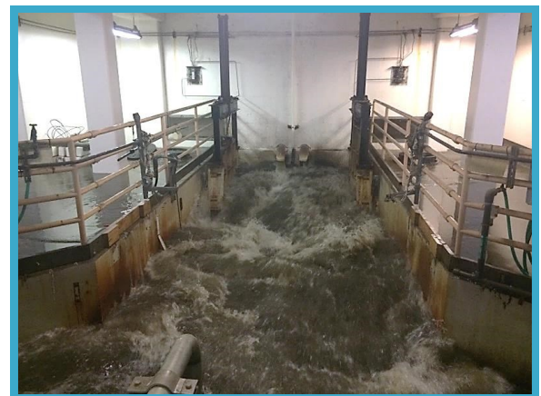
High channel levels caused by elevated influent flows from the Ross Valley and San Rafael interceptors.
