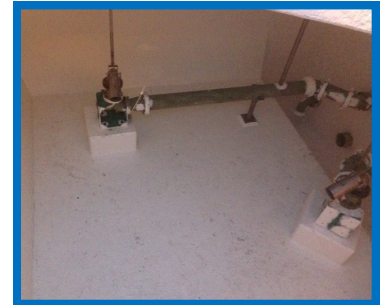
Vault with new epoxy coating.
