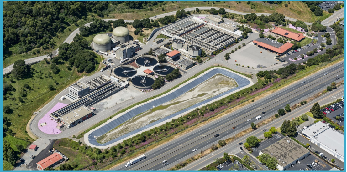
Aerial view of Agency facilities adjacent to Highway 580 in San Rafael.
