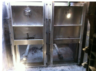
New influent channel gate.
