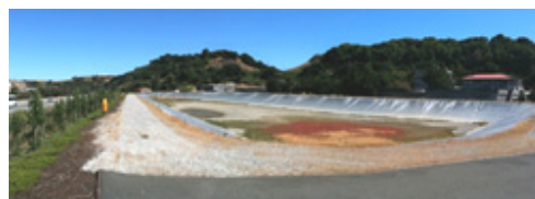
Effluent Storage Pond existing condition.
