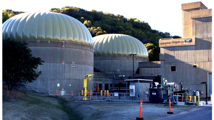
Digester membrane covers and FOG/F2E facility.
