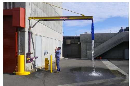
CMSA's recycled water delivery facility.
