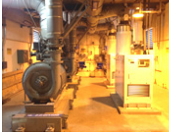
Old blowers on left remain as backup.
