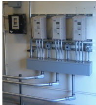
New feed pump controls.
