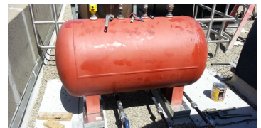
New installed tank.
