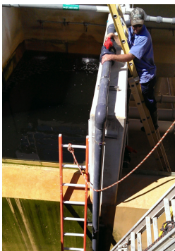
Temporary diffuser removal.
