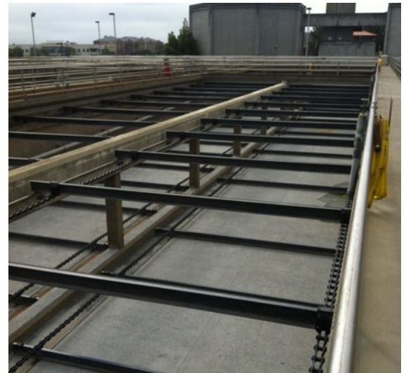
View of rehabilitated Primary Clarifier No. 3.
