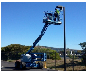
Staff retrofitting a fixture in place.
