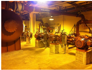
New pumps, strainer and tank.
