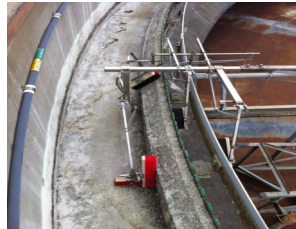
New brushes in place.
