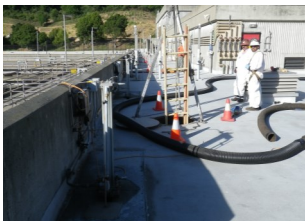
Grit being removed with an industrial vacuum hose.
