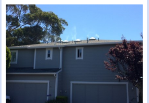
Smoke visible from roof vents.
