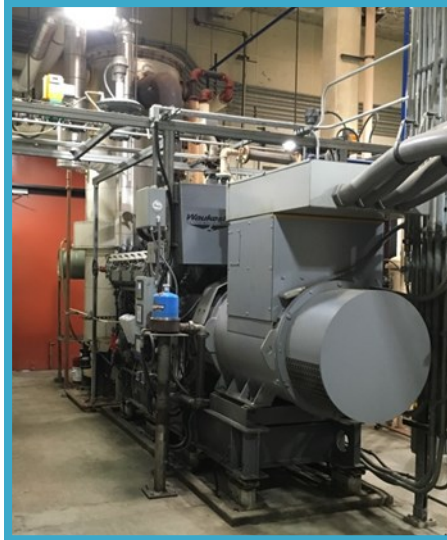
Existing cogeneration engine (left), and PG&E transformer and main plant switchgear (below).
