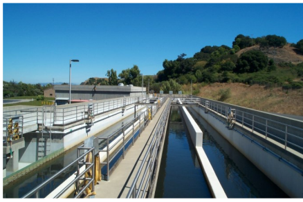
Chlorine Contact Tanks.
