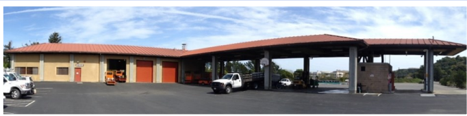
Existing Maintenance Building.
