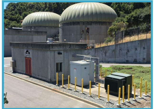
Existing cogeneration engine (left), and PG&E transformer and main plant switchgear (below).
