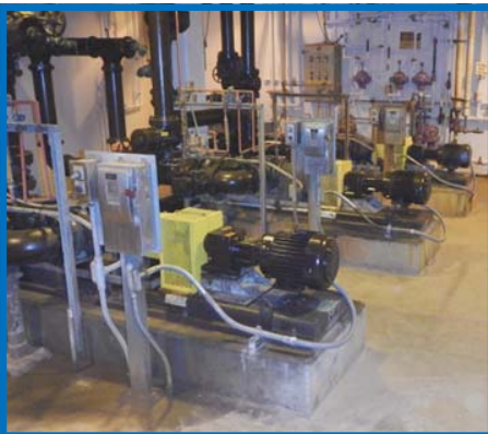
New centrifuge-feed pumps.
