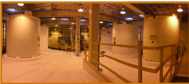
Existing hypochlorite storage room floor.
