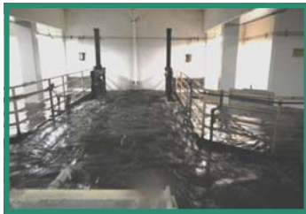
Headworks during the peak of the storm.
