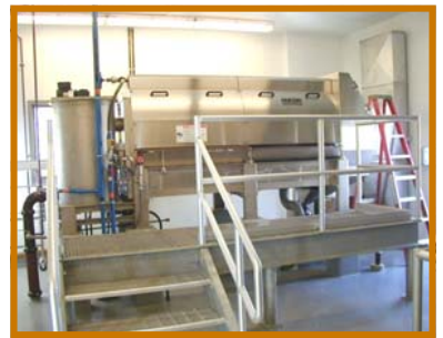
Example of rotary drum thickener (RDT).
