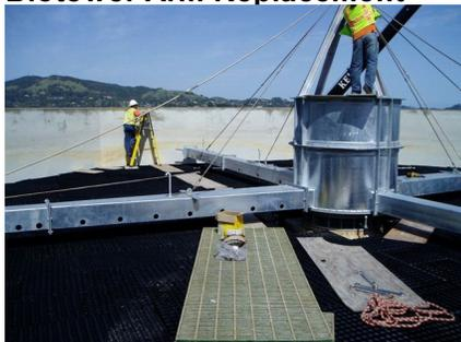
The new biotower equipment from Case-Cotter has been received. The Case-Cotter factory assembled the new stationary base, Agency-supplied replacement bearing, new turntable, and the first tier of the rotating tower. The contractor field-assembled the rest of the rotating tower together with the four biotower arms, and lifted the assembly 40-feet up to the top of the biotower.
