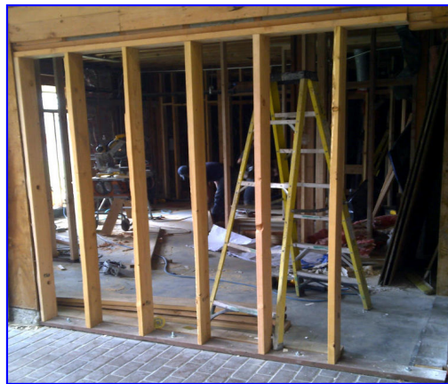
Wall framing of the women's locker room.
