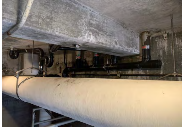
New ABS Drain Pipe
