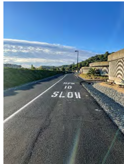
Main Road after slurry seal treatment and new pavement markings
