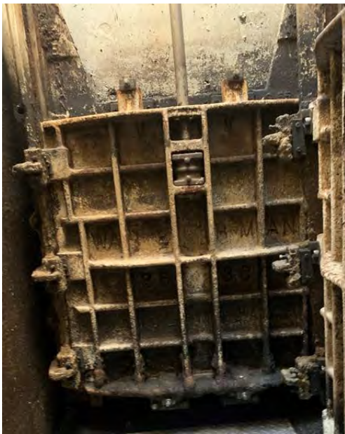
Originally installed cast iron sluice gate
