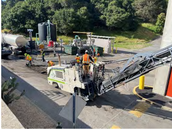
Grinding and spot repairing asphalt pavement by the Organic Waste Receiving Facility
