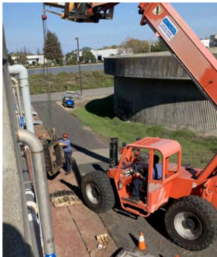
Using the Telehandler to position gates
