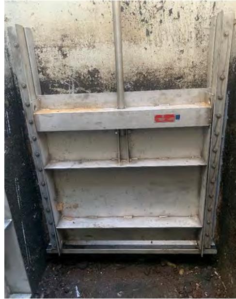
Recently installed stainless steel sluice gate
