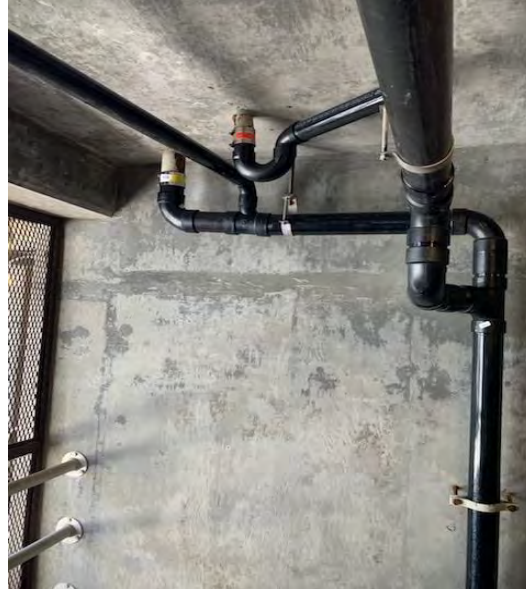
New ABS Drain Pipe
