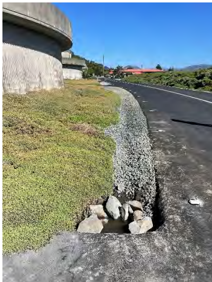
Regraded Drainage ditch by the recycle water fill station
