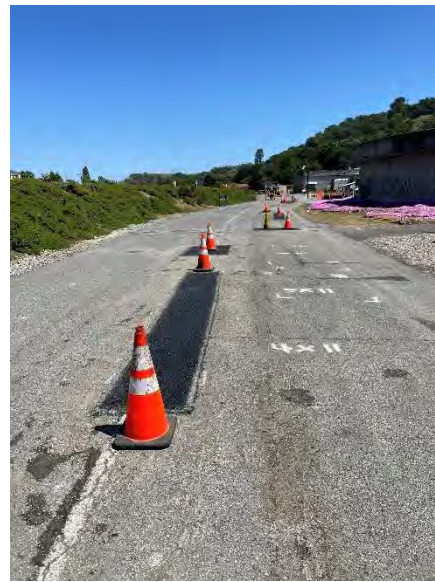
Spot repaired damaged road
