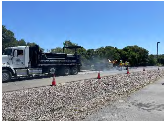
Repaving asphalt concrete
