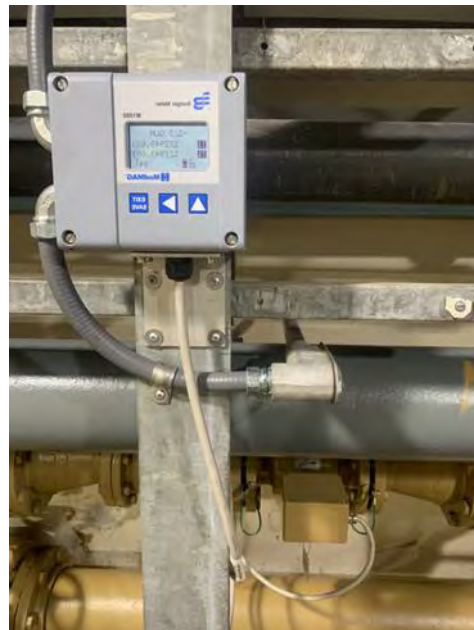
Controller for Sludge Flow Meters
