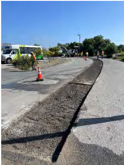
Removed section of damaged asphalt surfaces
