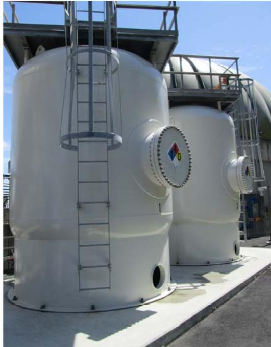
The effluent from the H<sub>2</sub>S removal system goes through a condenser to reduce moisture content before fed to two activated carbon adsorbers (Model SAG 48V, Applied Filter Technologies, Snohomish, WA) for siloxanes removal. The system consists of two vessels filled with GAC and operates in parallel and in an up-flow mode. Figure 3.9 is a photo of the siloxanes removal system. Some of the system parameters are listed below:
