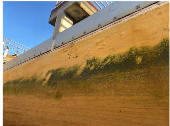
Figure 2: Failed Chlorine Contact Tank 4 coating
