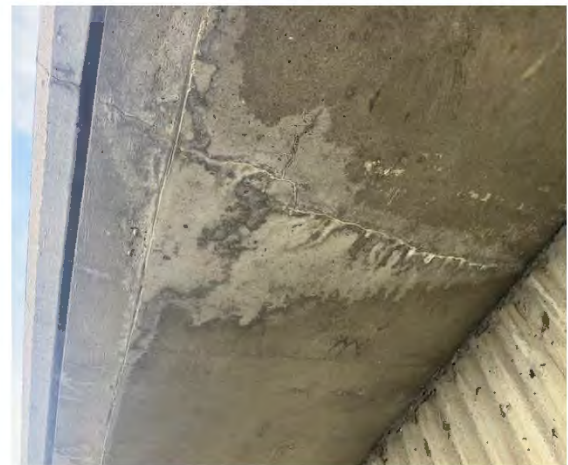
Figure 5: Signs of water seeping through walkway
