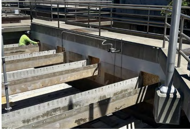
Figure 1: Recoating PC1 effluent through
