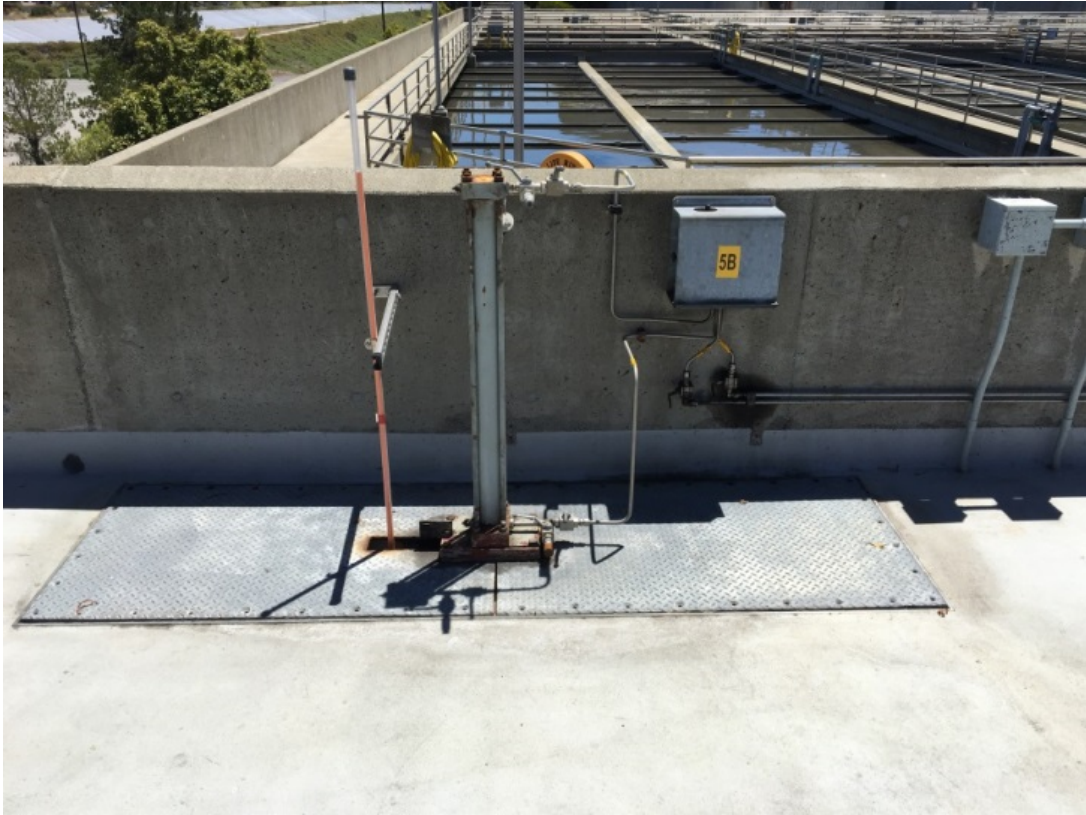
Photo 1 - Existing hydraulic gate operator on Primary Clarifier #5
