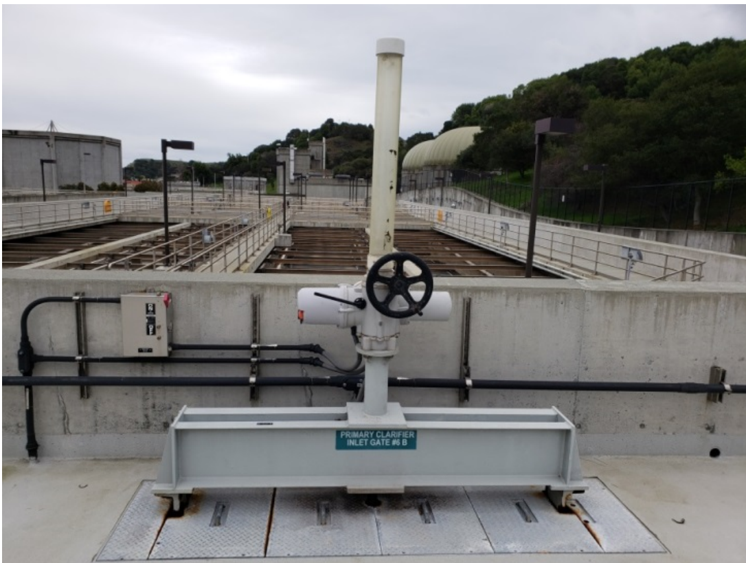
Photo 2 - Motorized gate operator on Primary Clarifier #6
