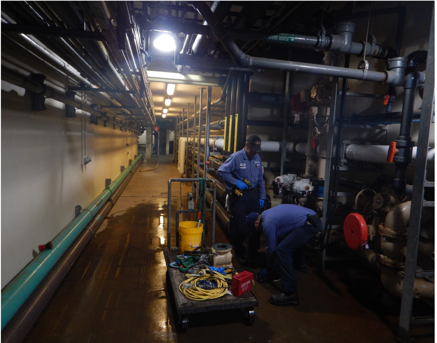
Agency technicians replacing a malfunctioning valve in the Solids Handling area
