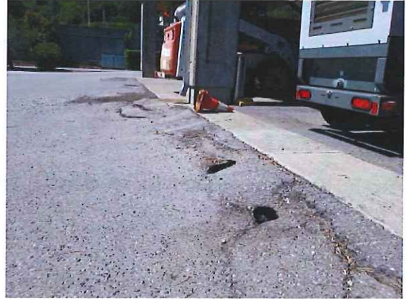
Sinkholes and pavement settlement along the Maintenance Building
