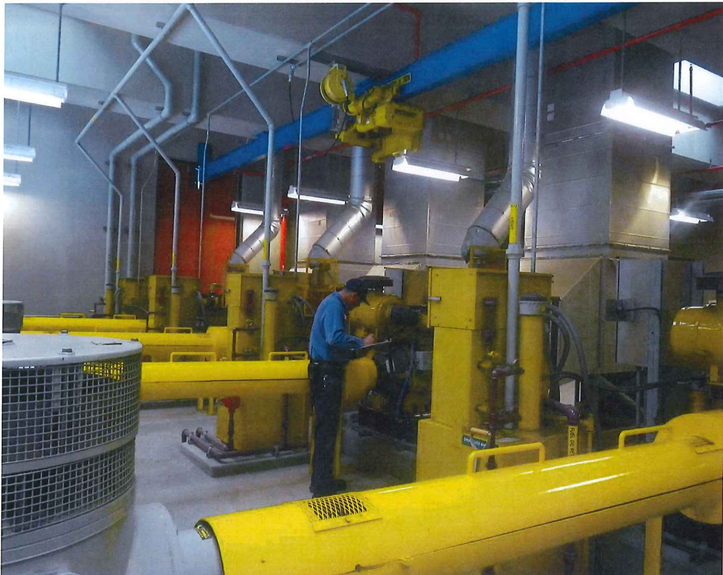
Technician A. Villarreal getting started on annual maintenance in the Effluent Pump Station.
