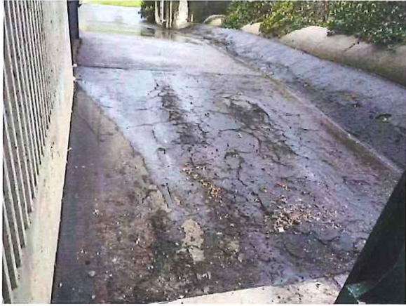
Asphalt pavement with cracks and potholes by the Ross Valley Interceptor
