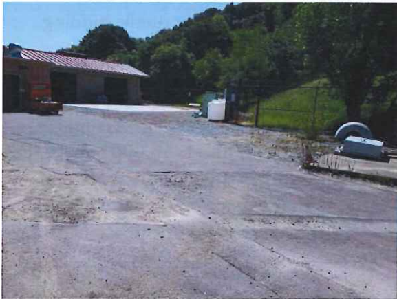
Gravel surfaces with drainage improvements needed by the Maintenance Annex
