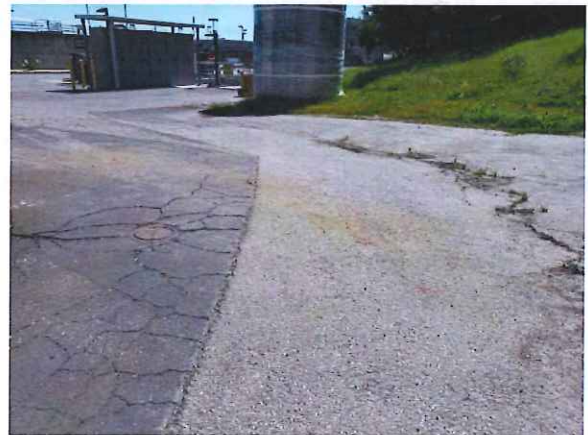
Excess wear and road pavement failure by the Solids Handling Building and Digesters
