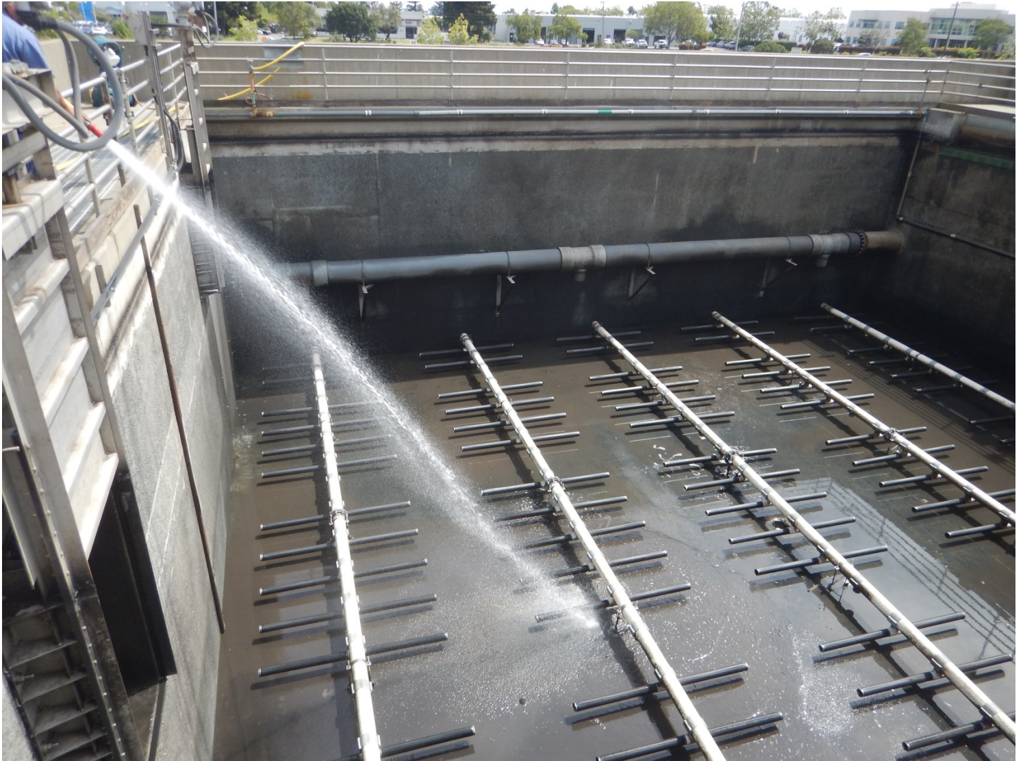
Aeration tank removed from service, and being cleaned and prepared for annual preventative maintenance.
