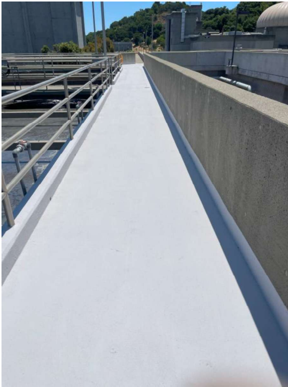
Photo 3: Newly coated primary clarifier deck.
