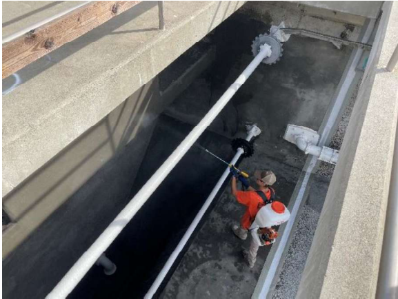
Photo 1: Applying waterproofing sealant to the resurfaced primary clarifier sludge hopper walls.
