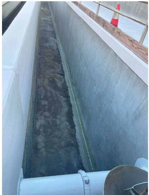
Photo 4: Fully rehabilitated chlorine contact tank (CCT) No. 4.
