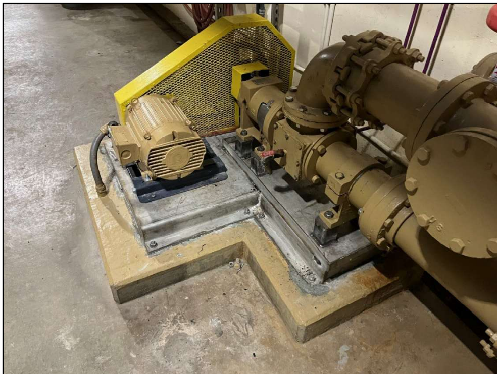
AFTER: New Primary Clarifier Sludge Stainless-Steel Motor and Pump Base
