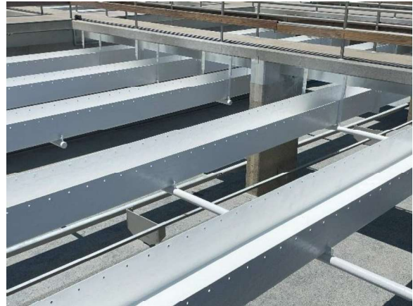
Photo 2: Recoated steel launder mechanisms.
