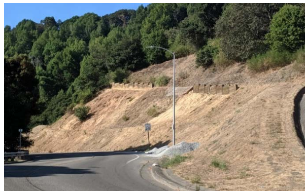
Landslides near front entrance (after)
