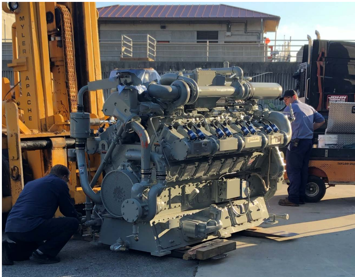
Cogeneration engine being unloaded and inspected prior to installation.
