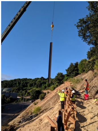
Contractor installing the I-beams
