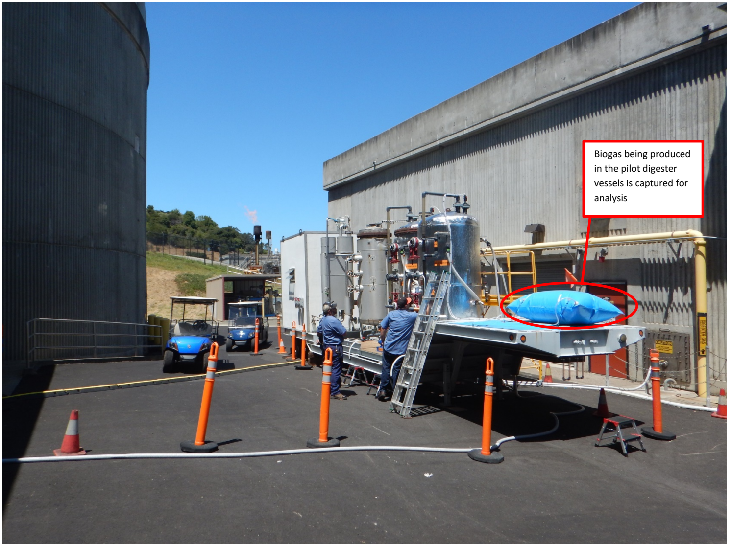
Pilot Digester System Technicians fine-tune equipment settings prior to full scale operation.
