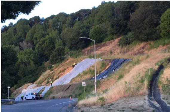
Landslides near front entrance (before)
