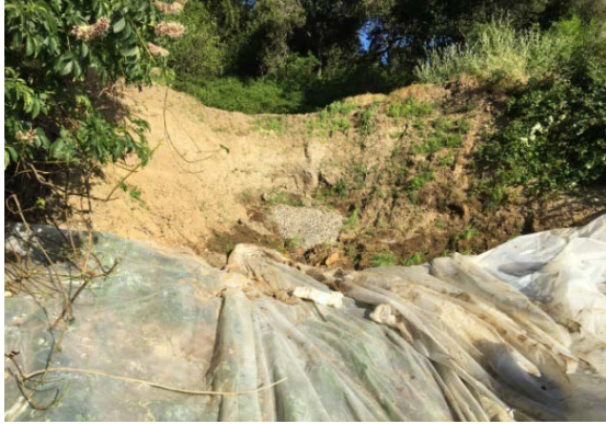
Biggest landslide near digesters (before)
