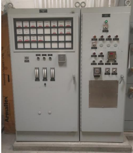
Existing Control Panel
