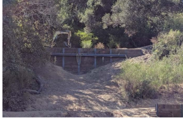
Biggest landslide near digesters (after)
