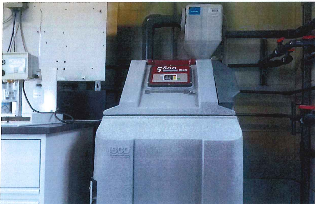
Facility effluent flow sampler installed in Decemeber
