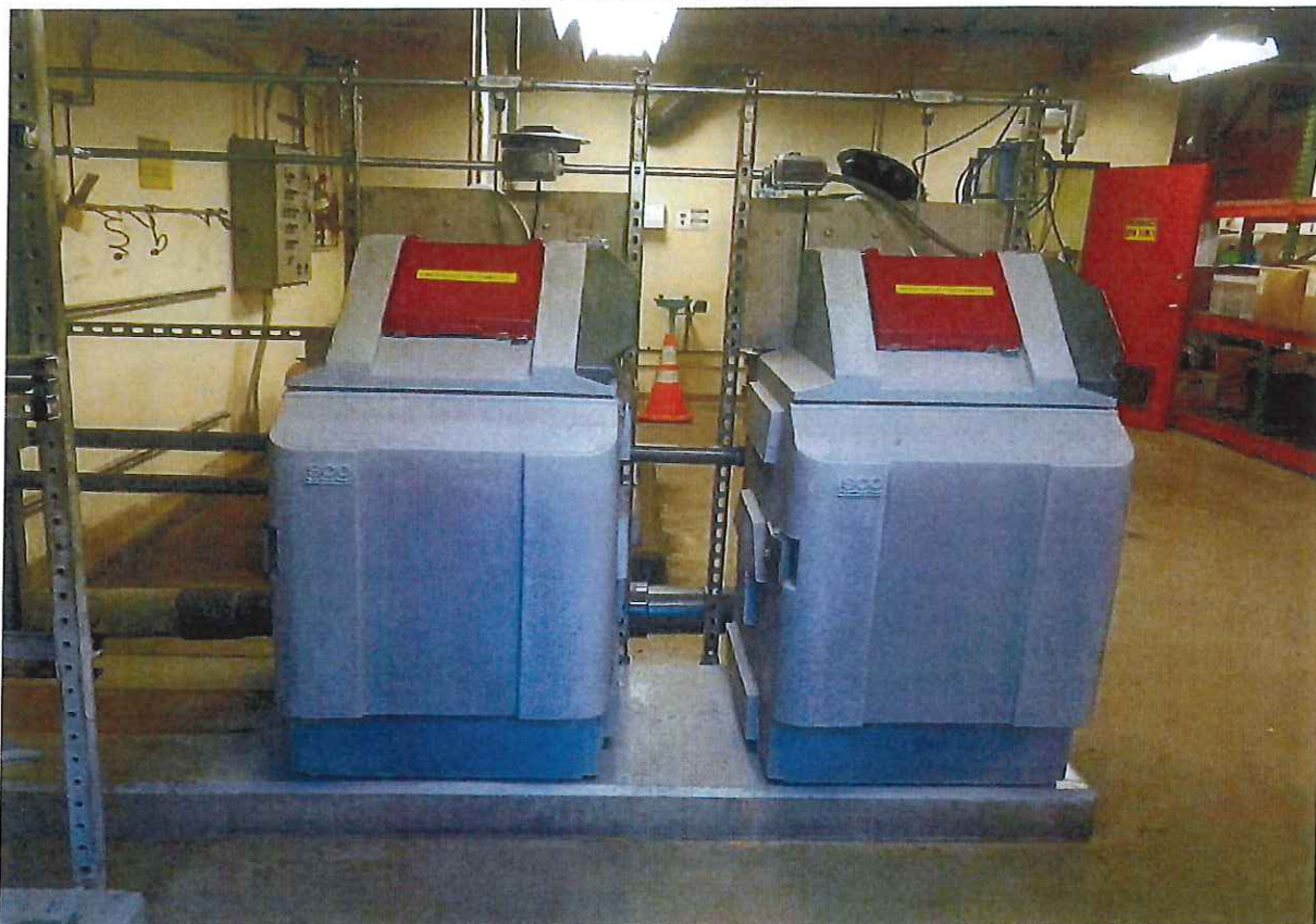
Facility influent flow samplers installed in November
