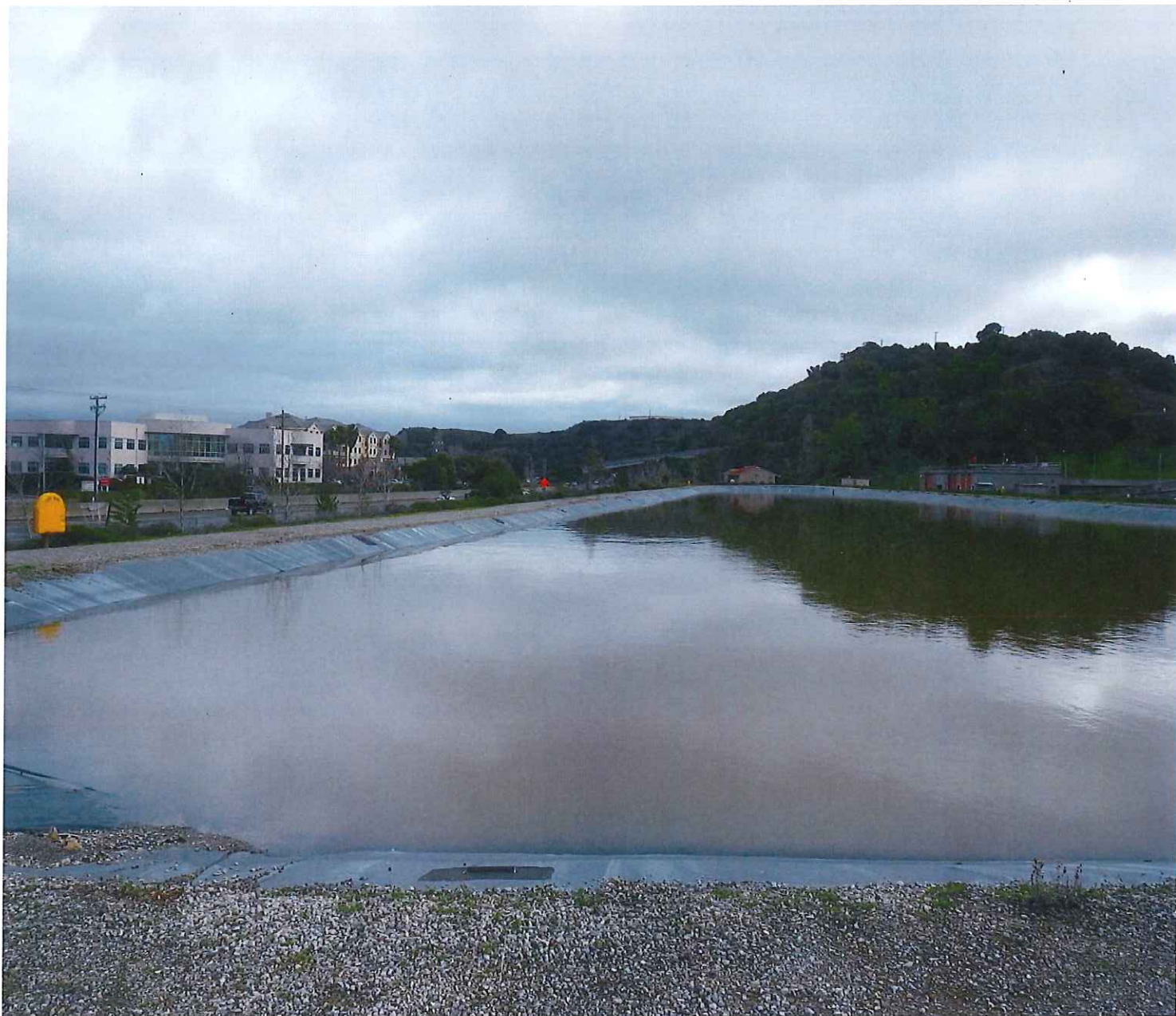
Effluent Storage Pond During the January 8 th Storm Event
