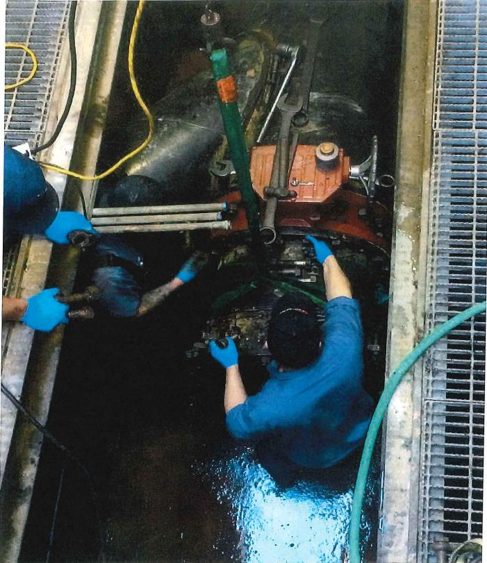
Technicians Replacing the Agency's Return Activated Sludge (RAS) Flow Meter
