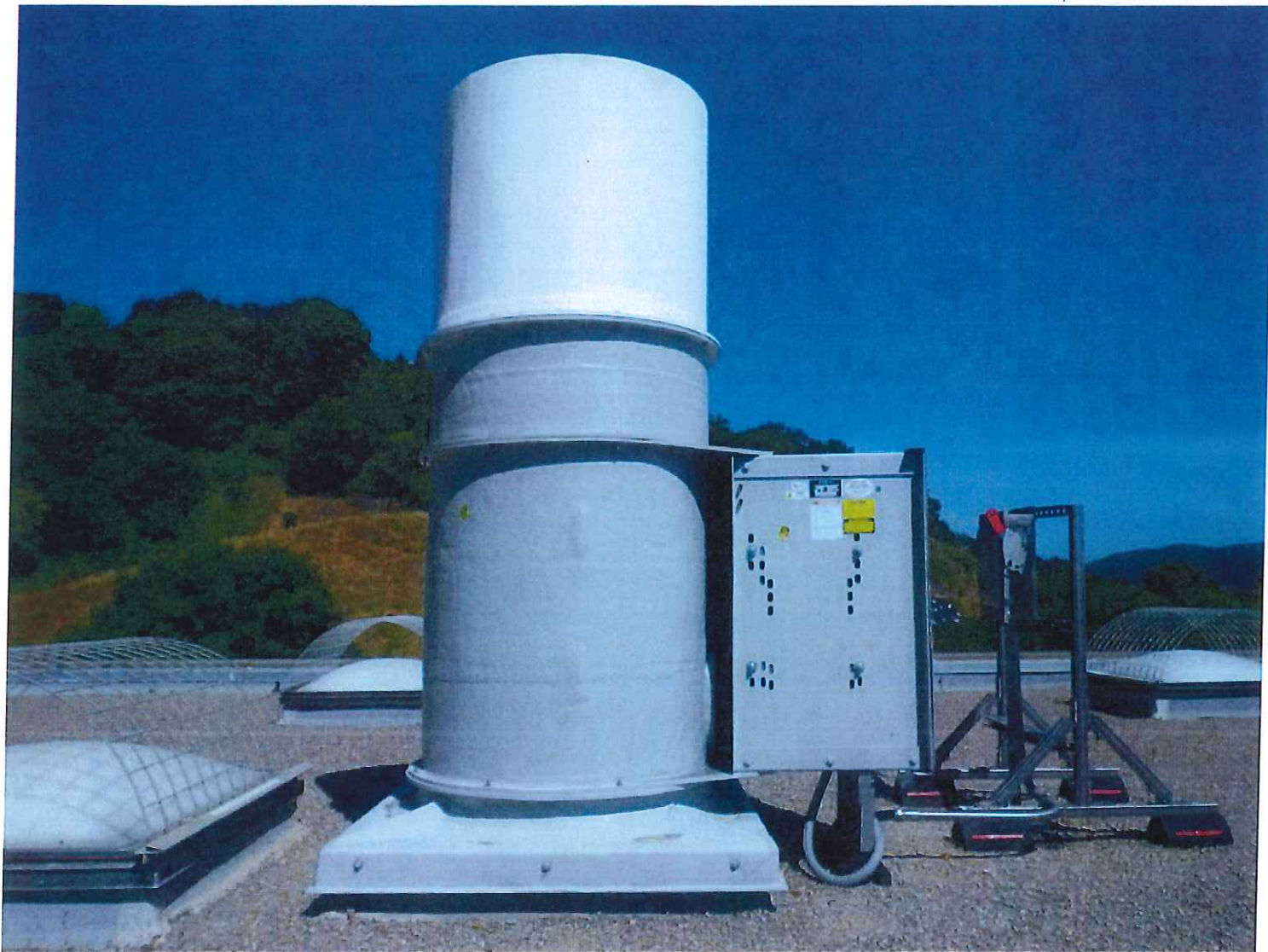
A new odor scrubber fan is mounted on the headwork's roof for ease of maintenance.
