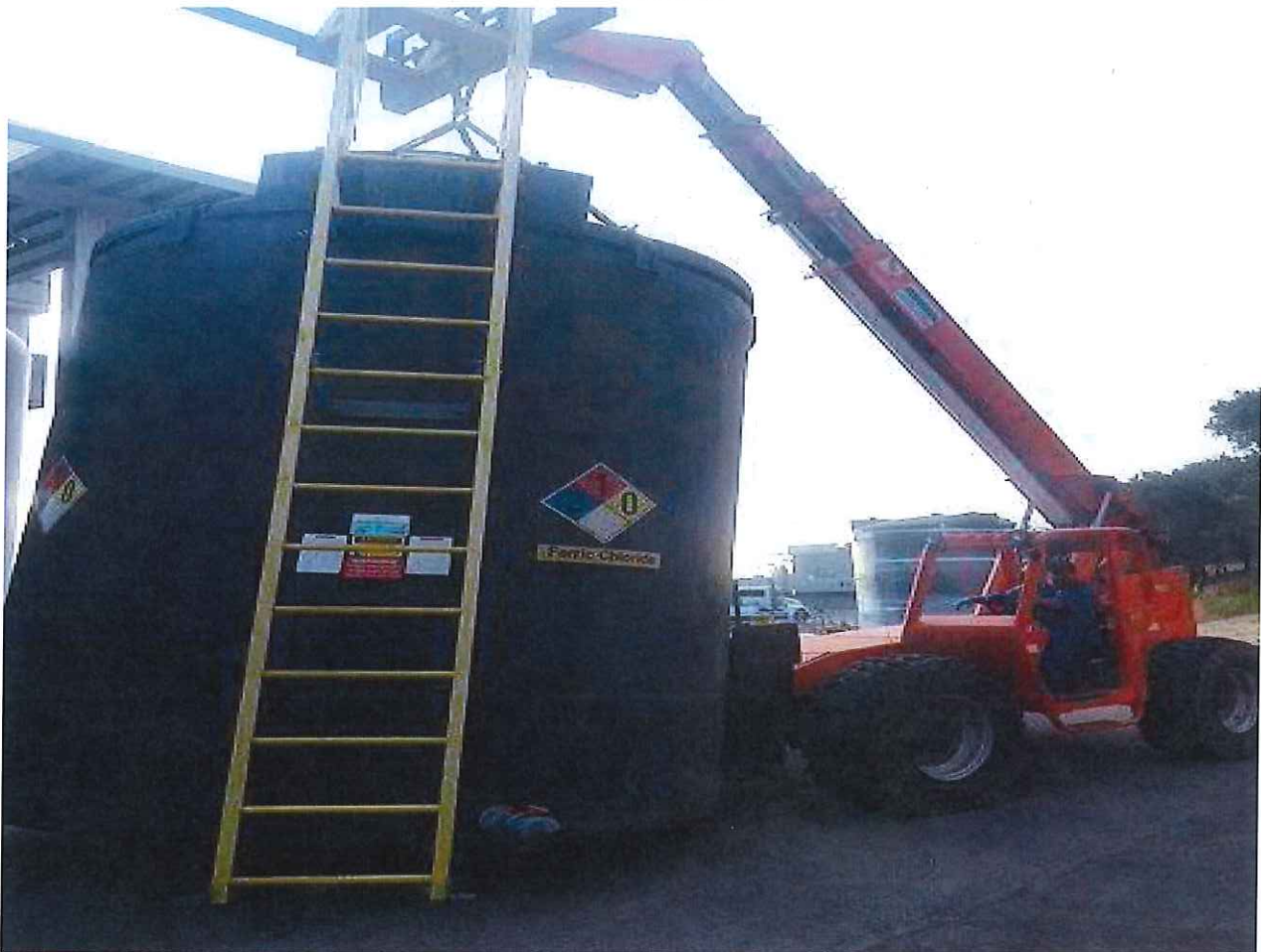
Agency personnel removing the original storage tank.
