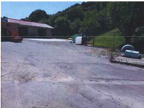
Photo 3 - Gravel surfaces with drainage improvements needed by the Maintenance Annex
