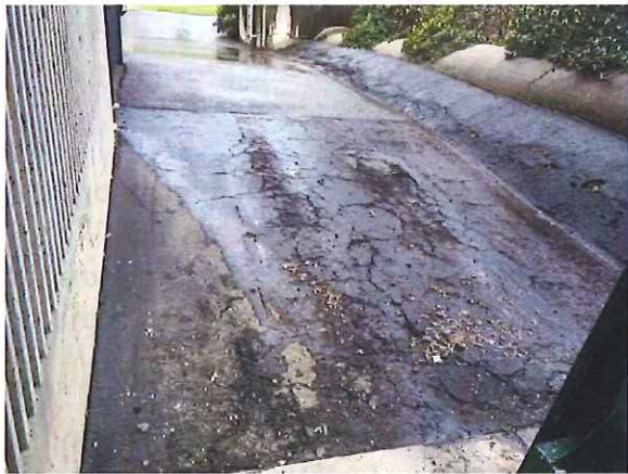
Photo 1 - Asphalt pavement with cracks and potholes by the Ross Valley Interceptor
