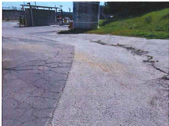
Photo 4 - Excess wear and road pavement failure by the Solids Handling Building and Digesters
