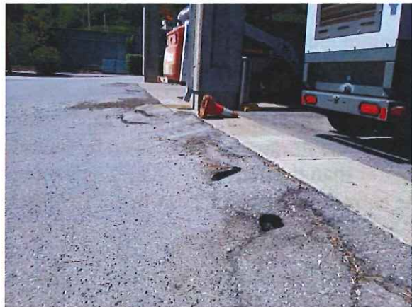
Photo 2 - Sinkholes and pavement settlement along the Maintenance Building
