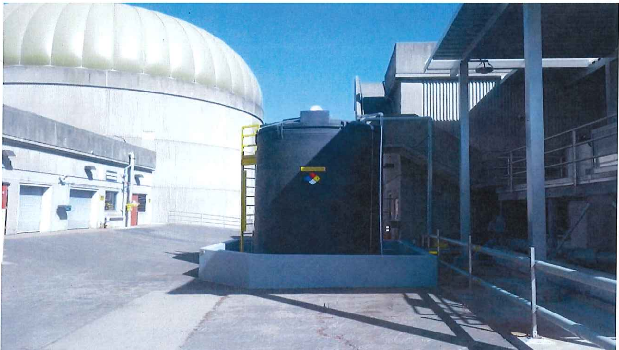
New storage tank installed and ready for use.
