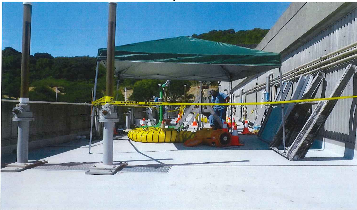
Staff performing a confined space entry to replace channel isolation gates under the influent channel deck.
