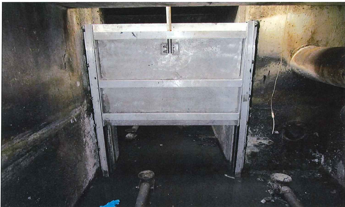
Recently installed influent channel isolation gate.
