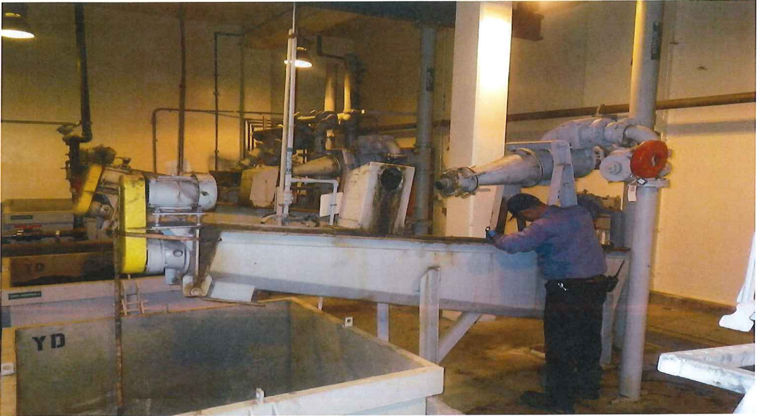
Maintenance Technician A. Villarreal performs annual preventative maintenance on a Grit Classifier.
