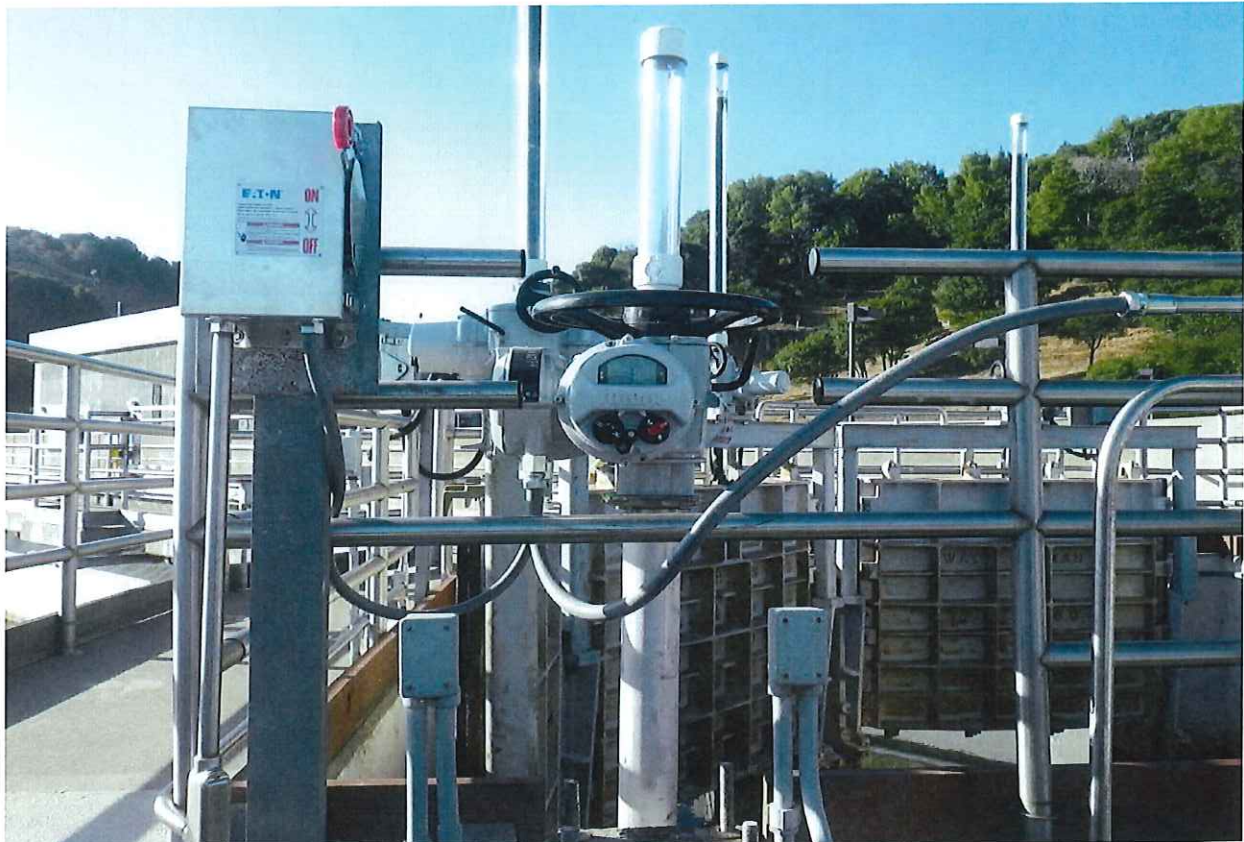
Newly installed automatic and SCADA controlled secondary effluent drain sump isolation gate.
