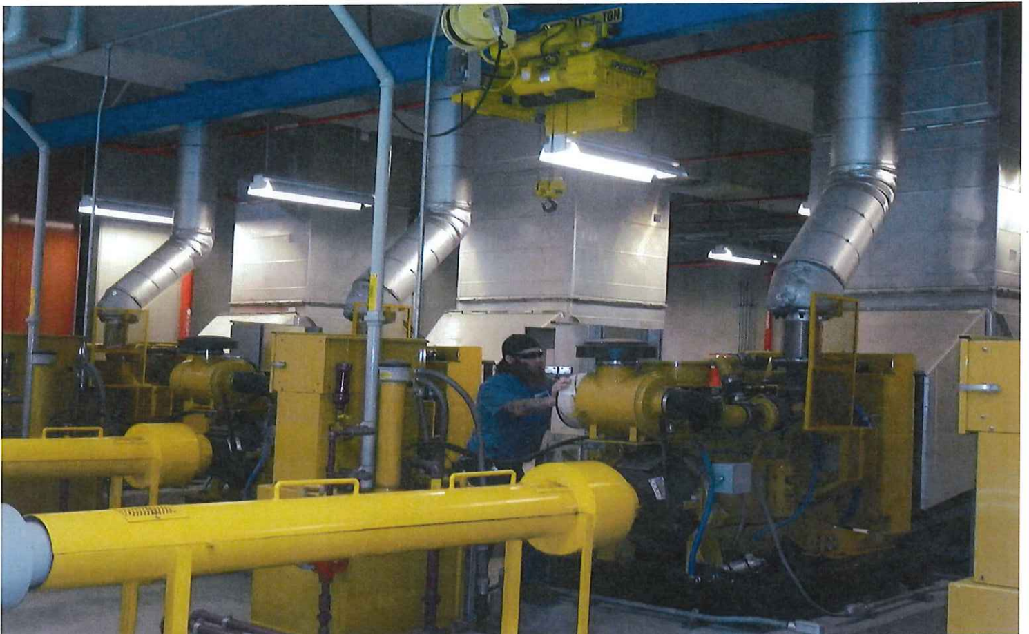
Maintenance Technician J. Clark inspects Effluent Pump Station pumps to confirm that they are ready for wet weather operation
