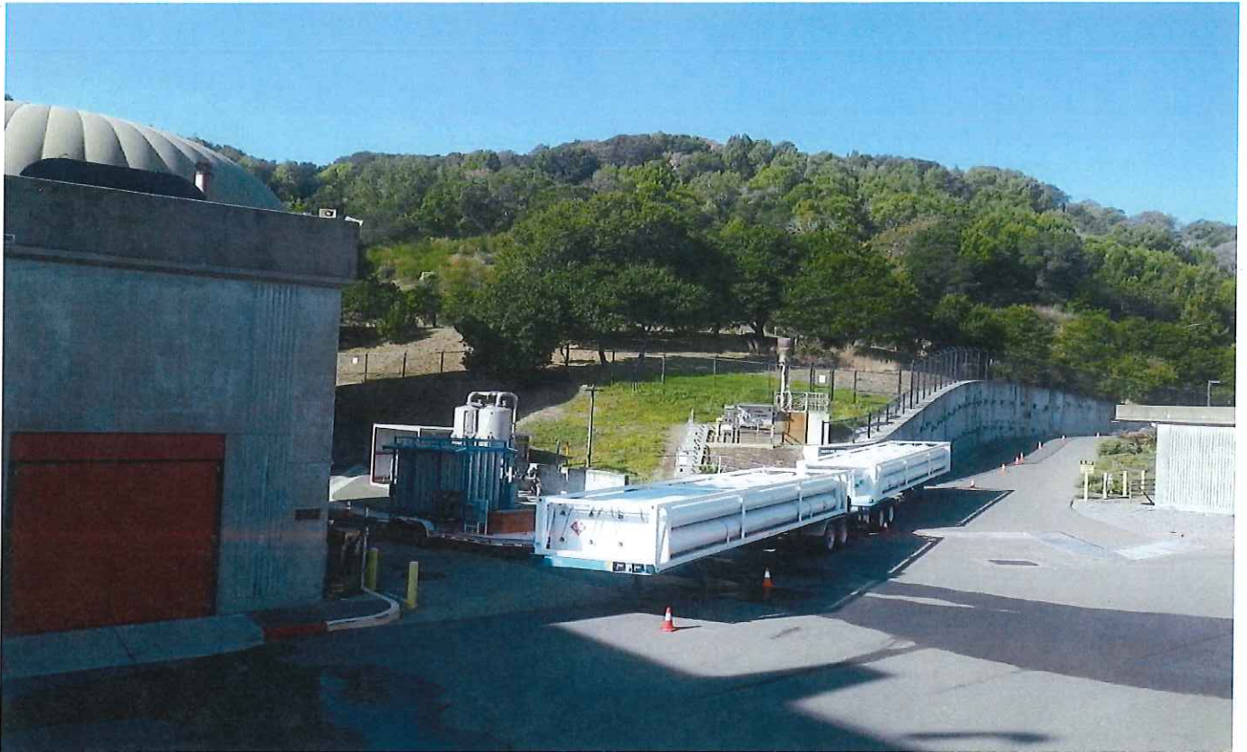
Cooperative work effort - PG&E uses CMSA site for natural gas injection into their distribution system via CMSA's NG piping.
