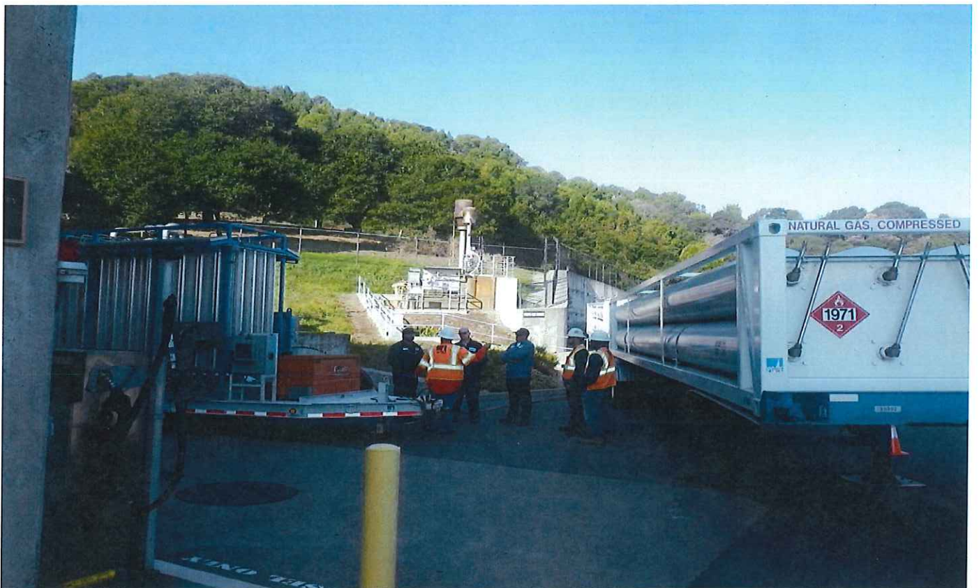
CMSA and PG&E technicians conduct a safety briefing prior to starting natural gas injection operations.
