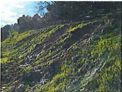
PHOTO 1: LANDSLIDE AT SITE 1
