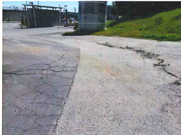
Excess wear and damaged road by the Digesters
