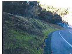
PHOTO 7: LANDSLIDE AT SITE 5
