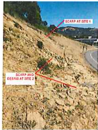
PHOTO 2: LANDSLIDES AT SITES 1 & 2
