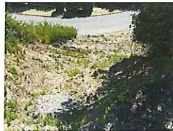
PHOTO 3: LANDSLIDE AT SITE 4 (LOOKING DOWN SLOPE FROM NEAR TOP OF SLIDE)
