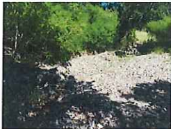
PHOTO 6: ACCESS ROAD AND EROSION ABOVE SLIDE AT SITE 4
