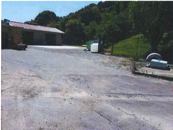
Compromised gravel surfaces by the Maintenance Annex
