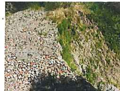
PHOTO 4: SCARP NEAR TOP OF LANDSLIDE AT SITE 4
