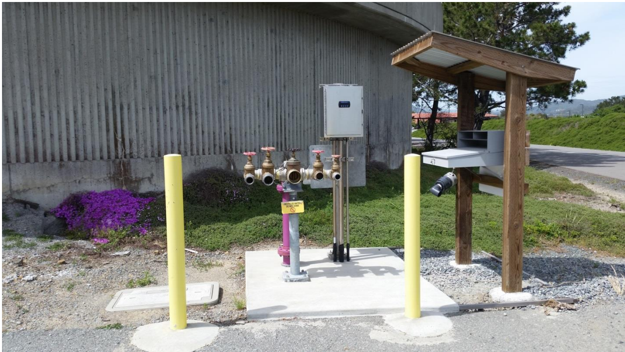
CMSA Recycled Water Truck Filling Station
