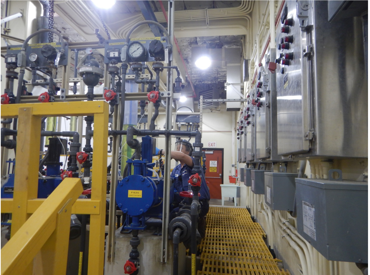
Operator A. Clark conducts performance testing on facility disinfection pumps in advance of an impending rain event.
