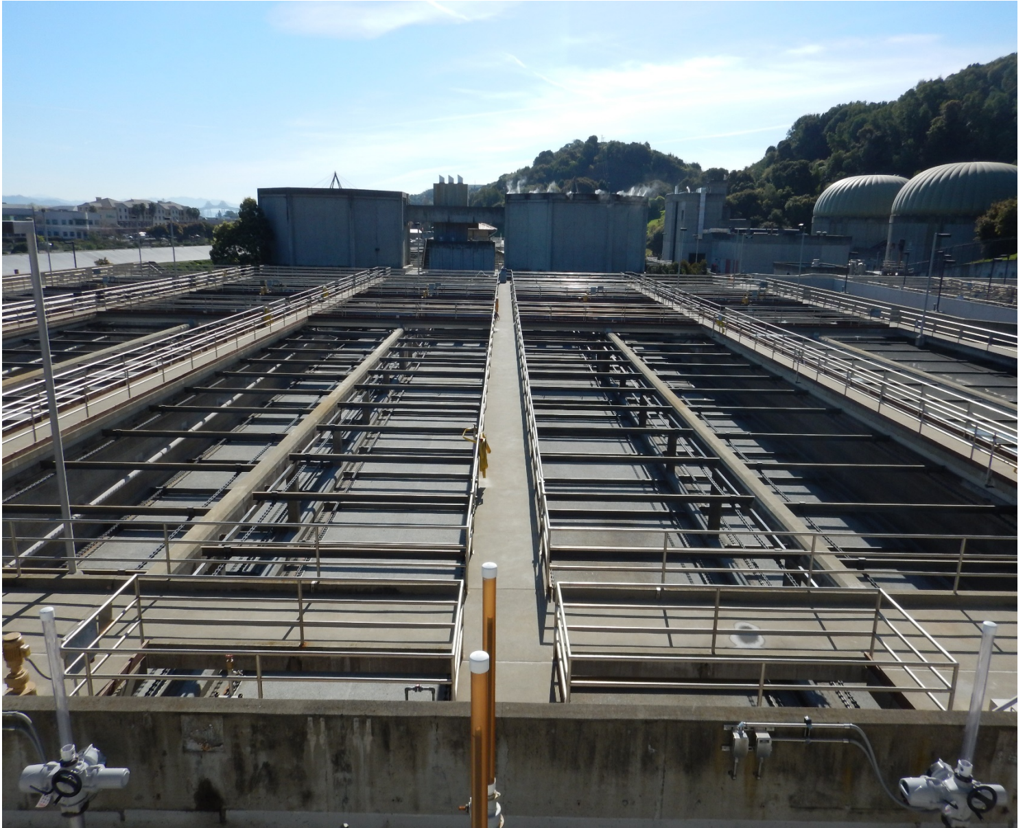
Process equipment offline as dry weather operations continue with no rain in February
