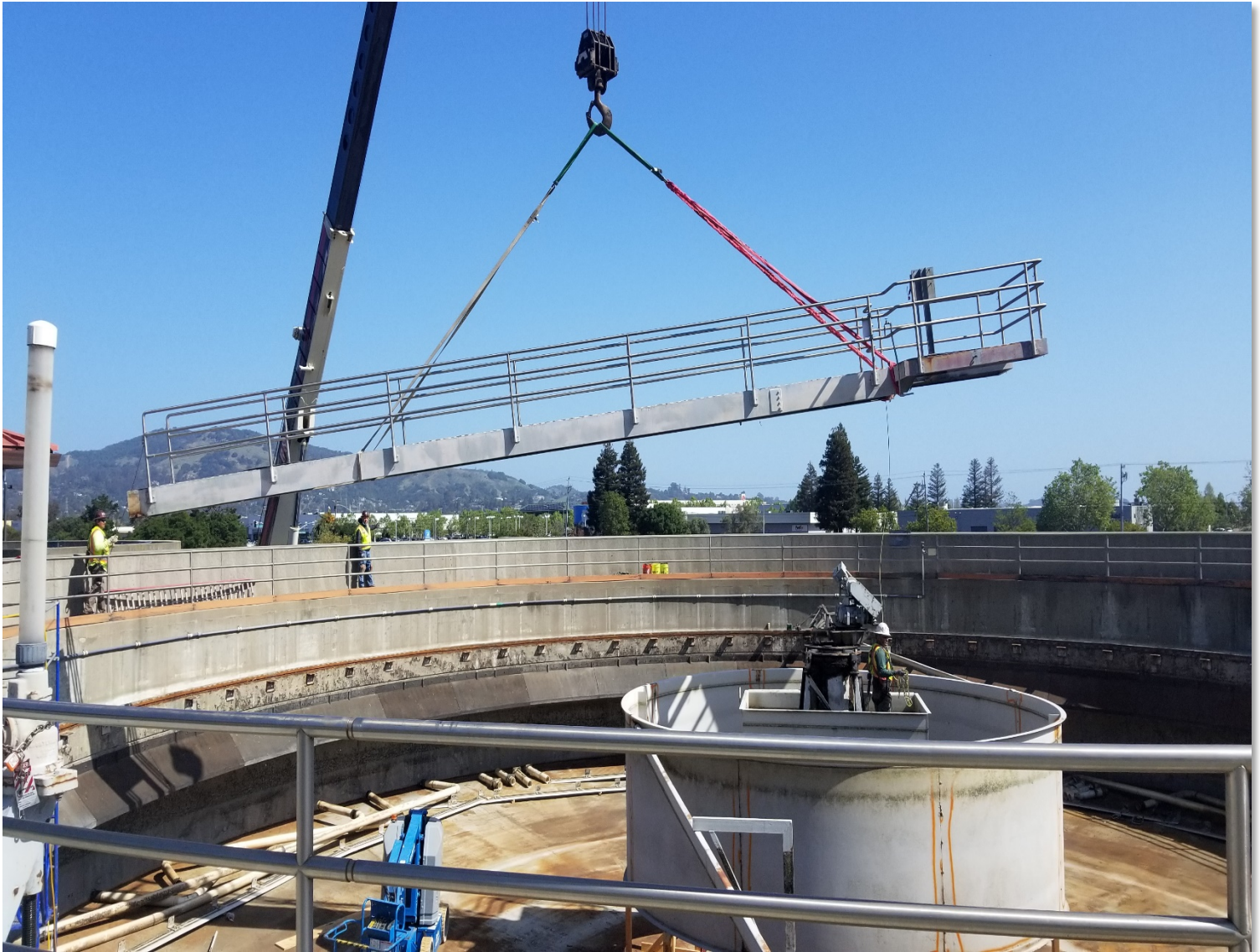
Contractors removing the center walkway from Secondary Clarifier No.3 as part of this clarifier's rehabilitation work.
