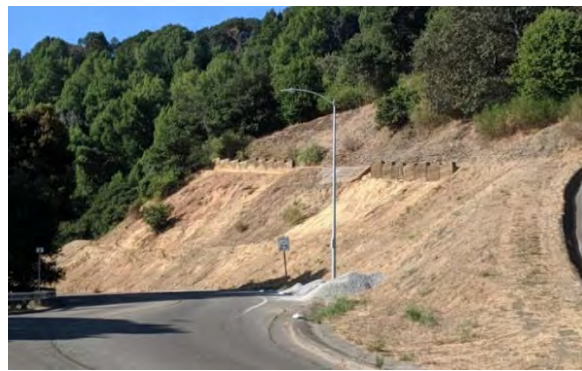
Landslides near front entrance (after)
