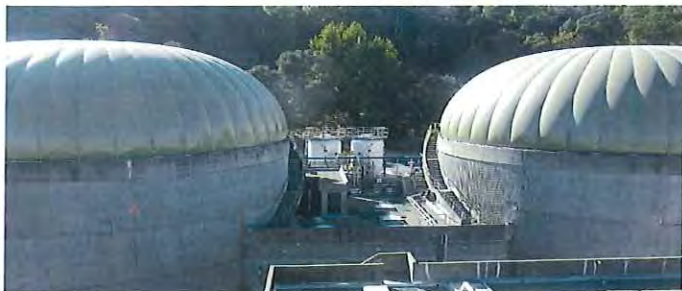
Anaerobic digesters with membrane covers
