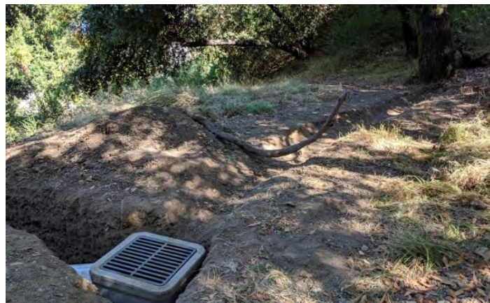
New swale and drop inlet behind the biggest landslide
