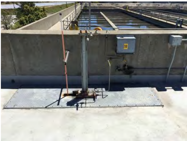
Old primary clarifier hydraulic gate.
