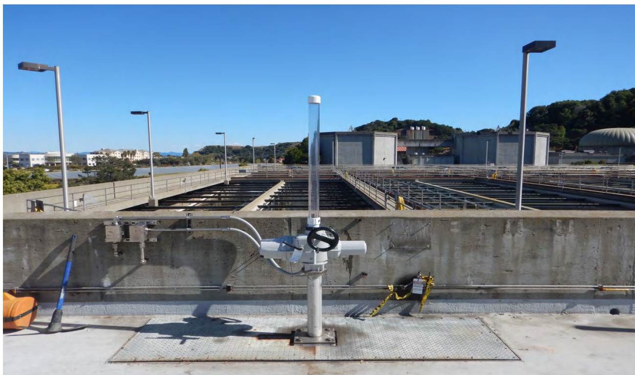
New primary influent motor operated gate.
