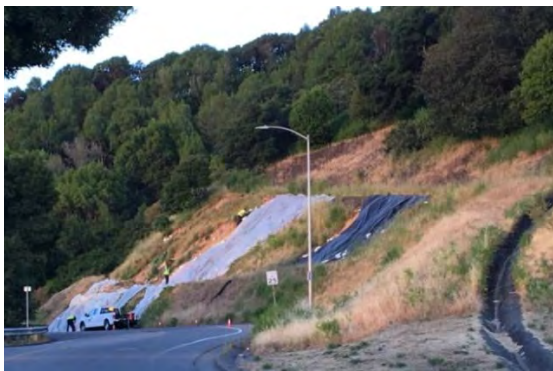
Landslides near front entrance (before)
