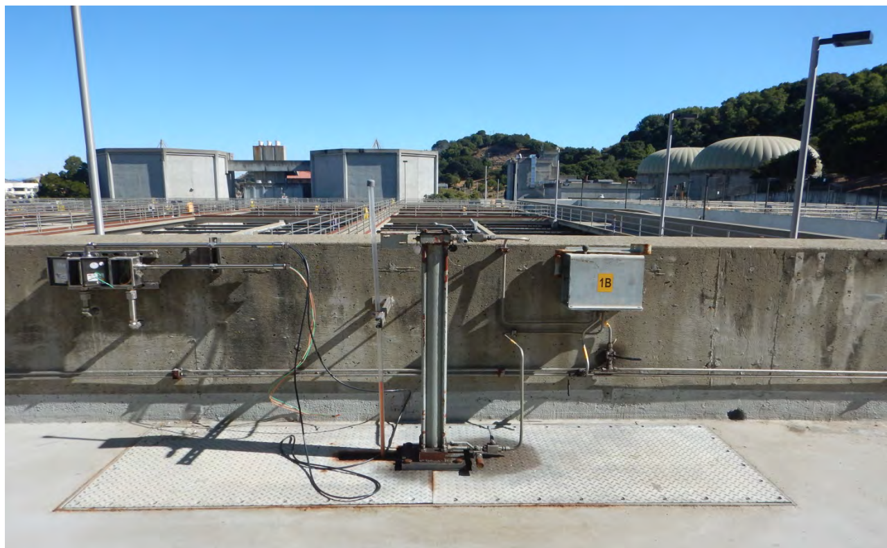
Old primary influent hydraulic gate.
