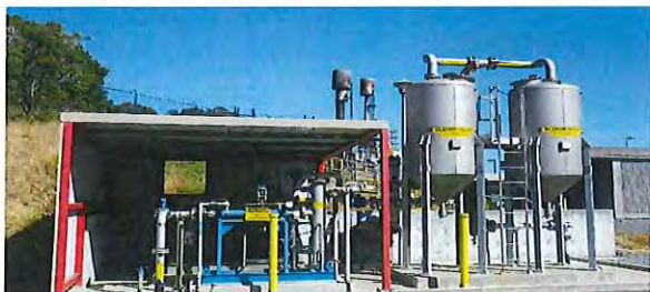
Biogas - moisture and siloxane removal
