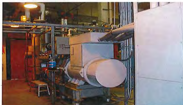
750 kW cogeneration system
