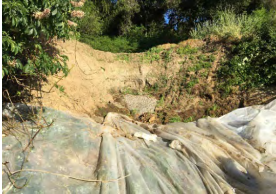
Biggest landslide near digesters (before)
