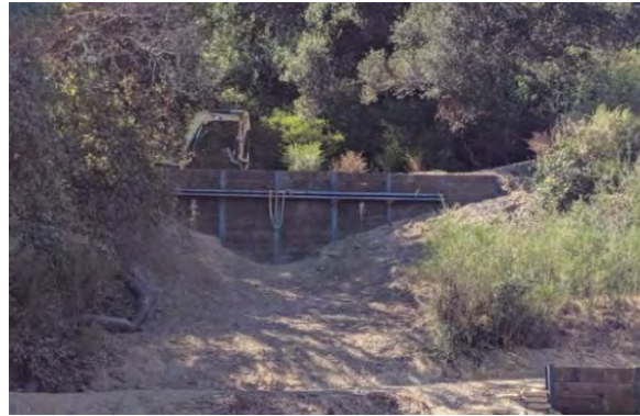
Biggest landslide near digesters (after)
