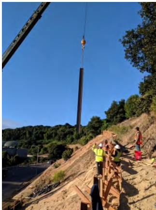
Contractor installing the I-beams
