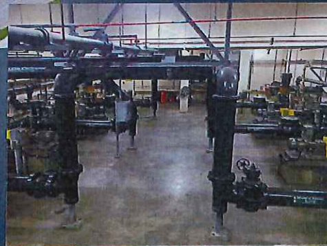
Secondary Clarifier Pump Room (RAS/WAS)
