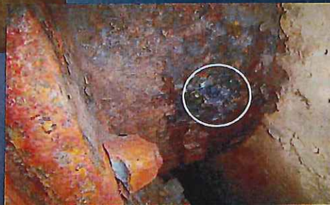
Pipes showed severe corrosion and minor leakage. The circled area is where only the mortar lining remained.
