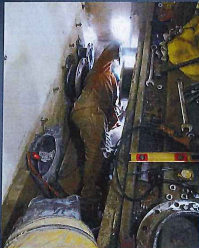
Field welding new flange couplings in a tight working space
