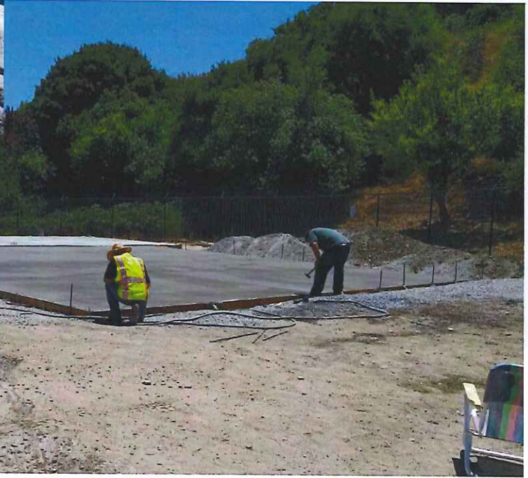
Foundation Slab and Approach Slab Concrete Pours
