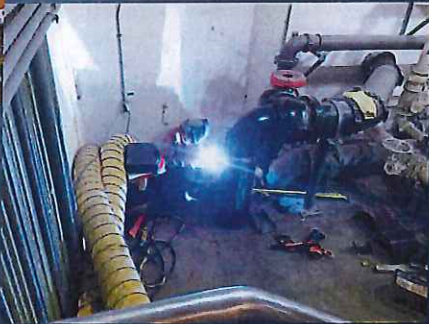
Field welding new steel pipes and flanges
