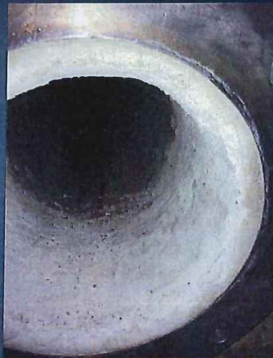
Applied new cement-mortar liner onto the steel pipe
