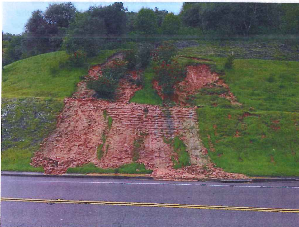
Landslide before debris removal
