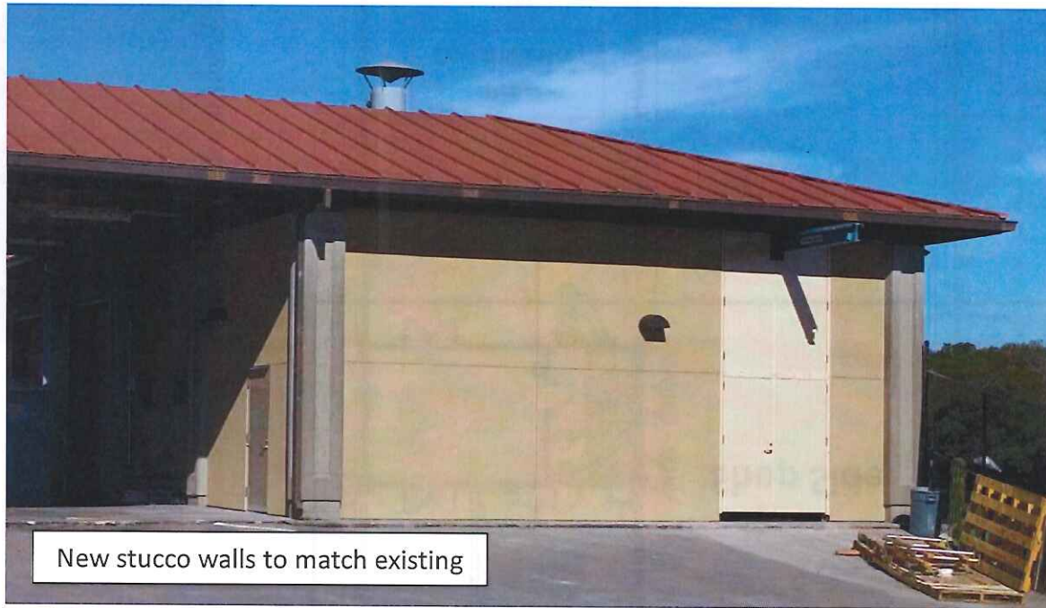
Newly Enclosed Shop of the Maintenance Building – Exterior View
