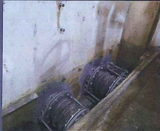
Completion of pipes repair with new pipe flanges, flexible couplings, grout, and protective coating
