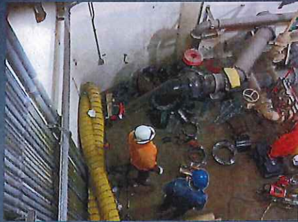
Contractor staging to perform pipe repairs
