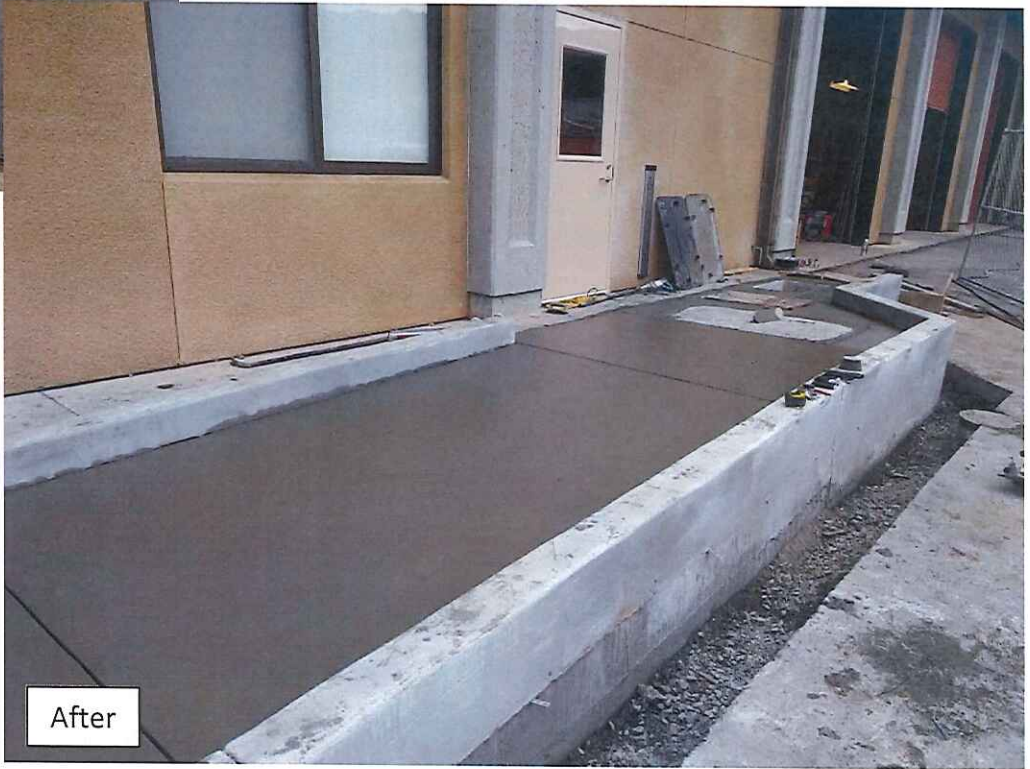
Ramp Access to Maintenance Building
