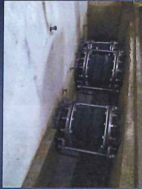
Installed new pipes and flexible couplings
