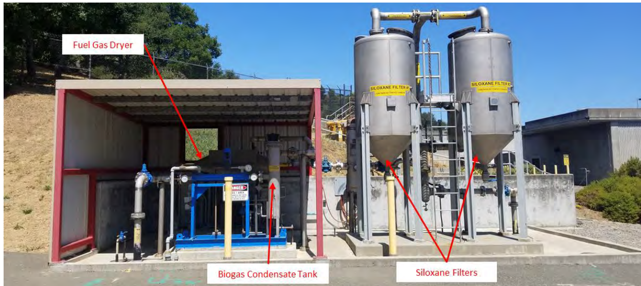
Photo 2: Existing Gas Treatment System
