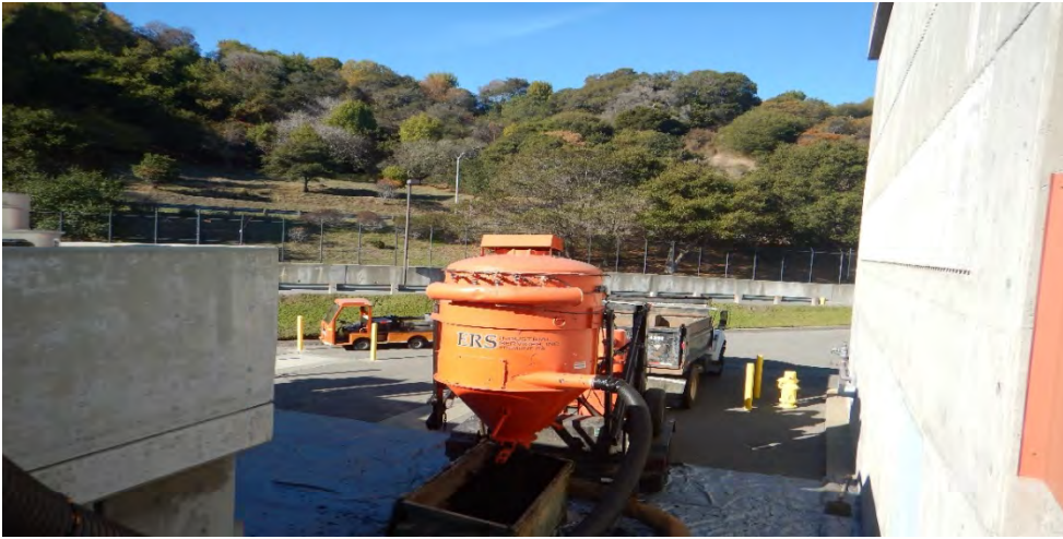
Picture 1: Staging equipment for the primary influent channel clean-up as part of the headworks channel blower efficiency study.
