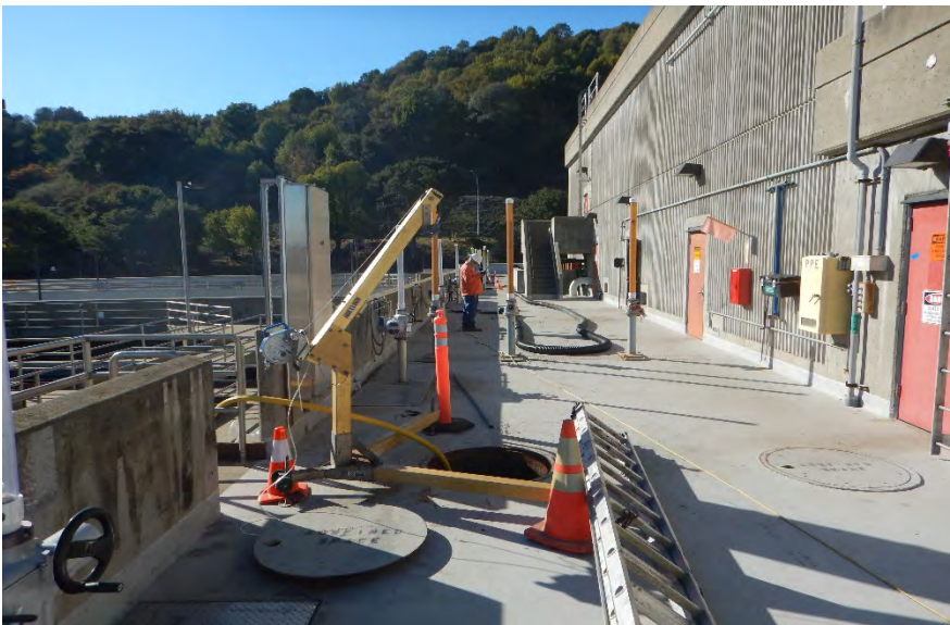
Picture 2: Contractors performing entry to clean the primary clarifier influent channel.
