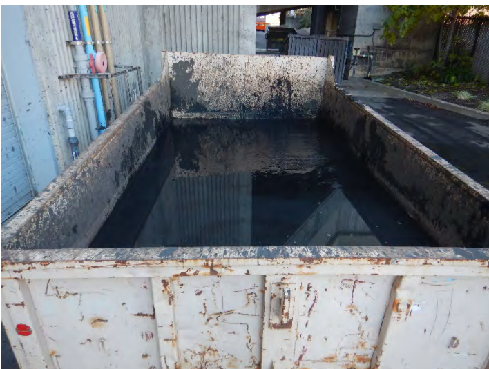
Picture 3: Grit / sand removed from the primary clarifier influent channel.
