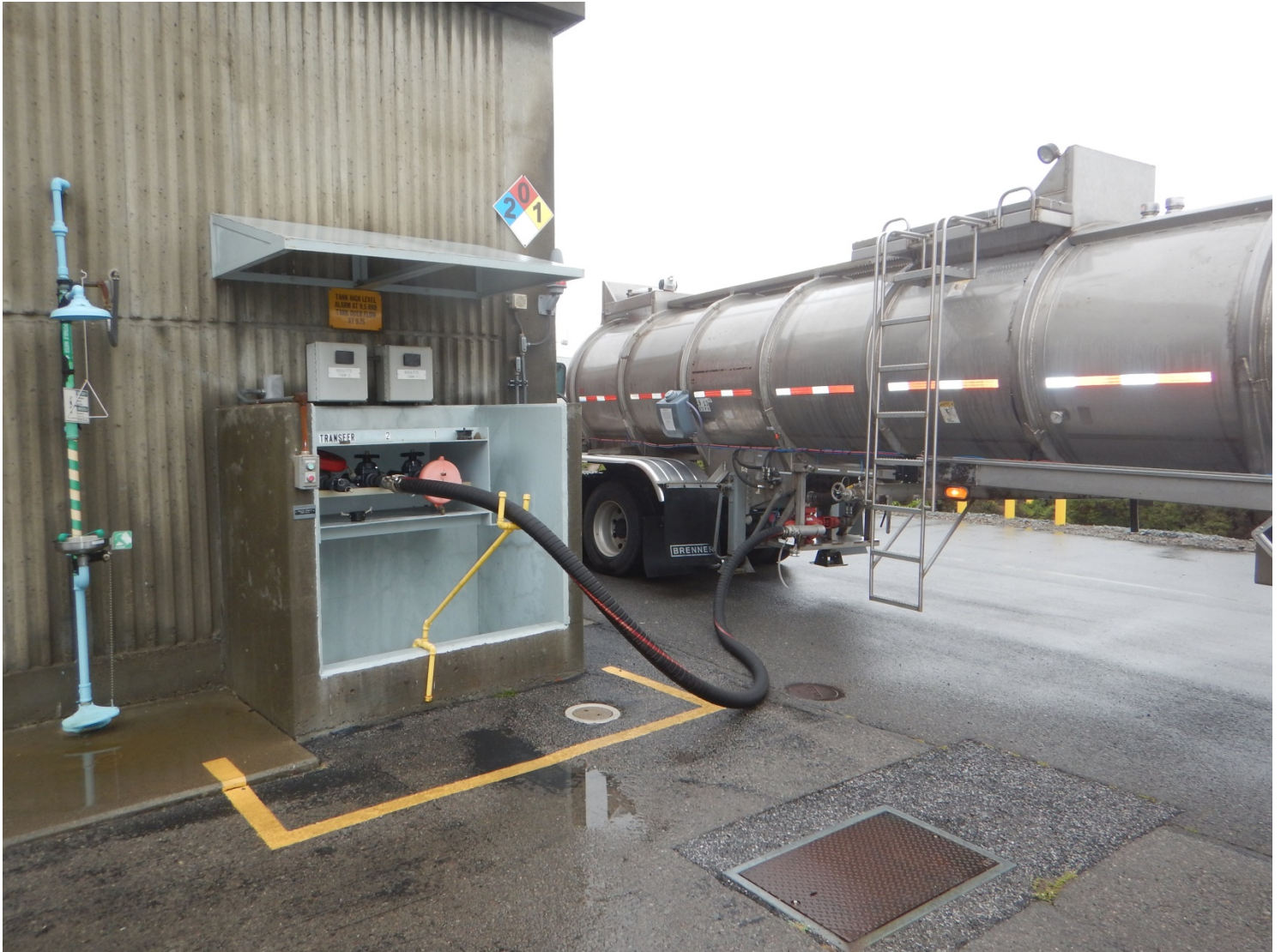
Receiving a delivery of Sodium Bisulfite Solution in preparation for the onset of a large storm event.
