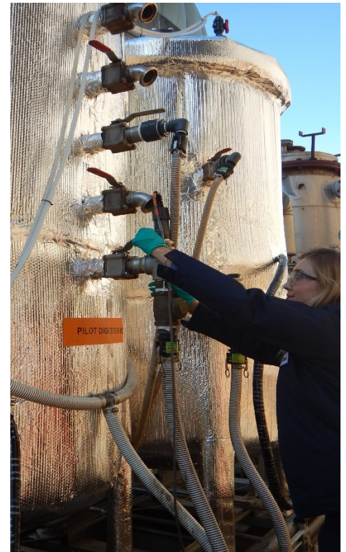
Operator Claire Ernst pouring “food” into a mixer prior to feeding this cuisine to the Pilot Digesters.
