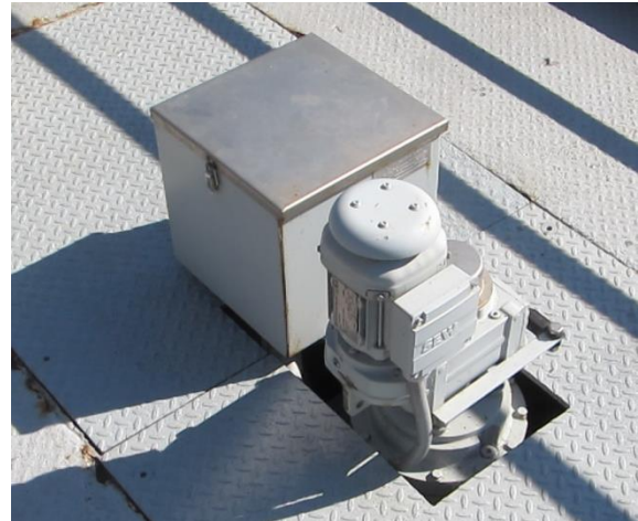
Current conditions of Secondary Clarifier No. 2 Drive (DBS unit installed in 2011)
