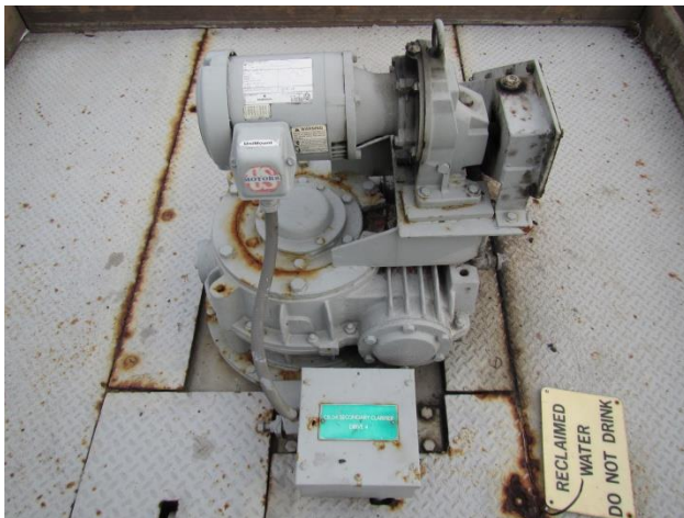
Current conditions of Secondary Clarifier No. 4 Drive (WesTech unit installed in 1985)
