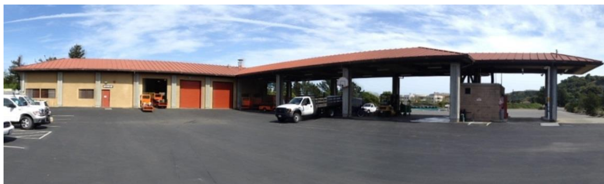
Maintenance Building with standing seam metal roofs.
