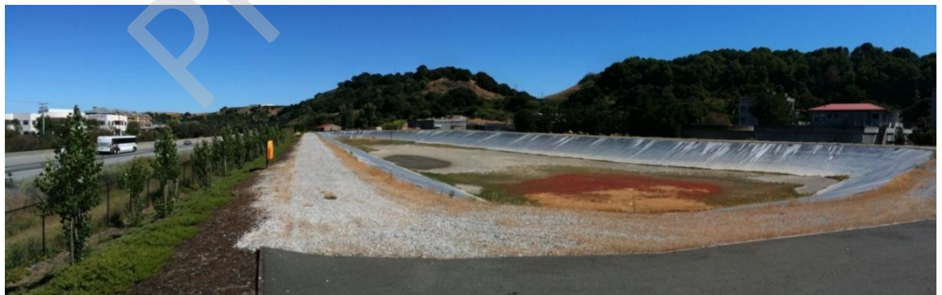
Effluent Storage Pond
