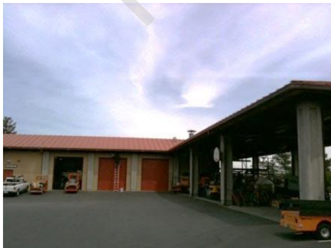
Maintenance Building and Covered Portico
