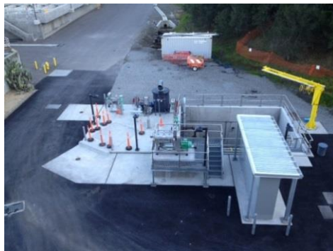
Organic Waste Receiving Facility
