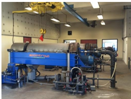
Existing Centrifuges
