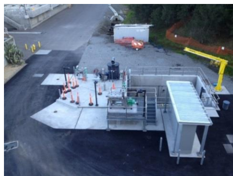
Organic Waste Receiving Facility
