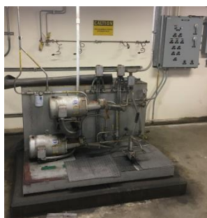
Hydraulic control system
