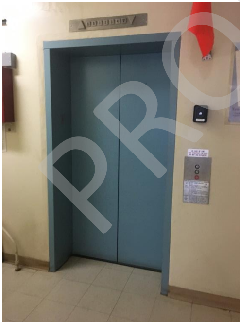
Solids Handling Building Elevator
