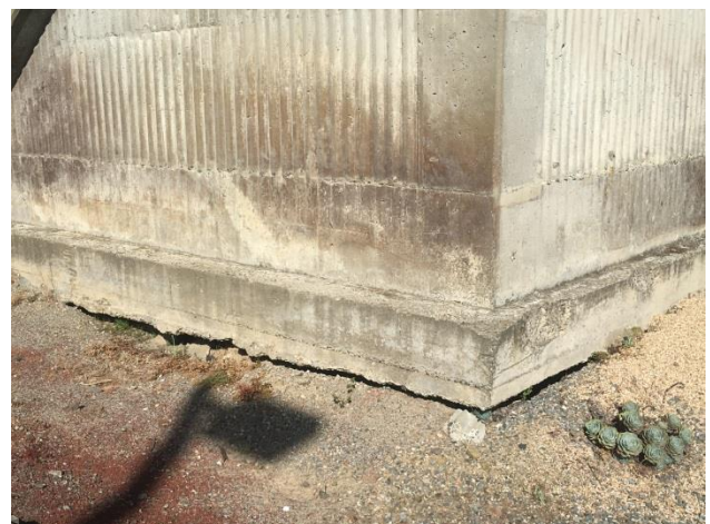
Exposed bottom of process tank
