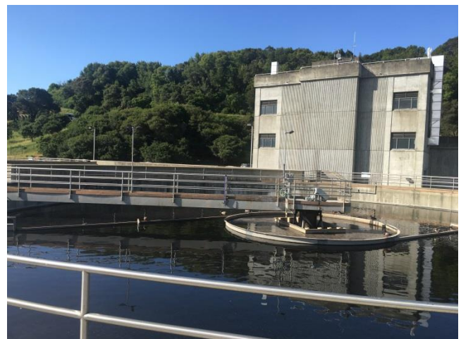
Secondary clarifier in operation
