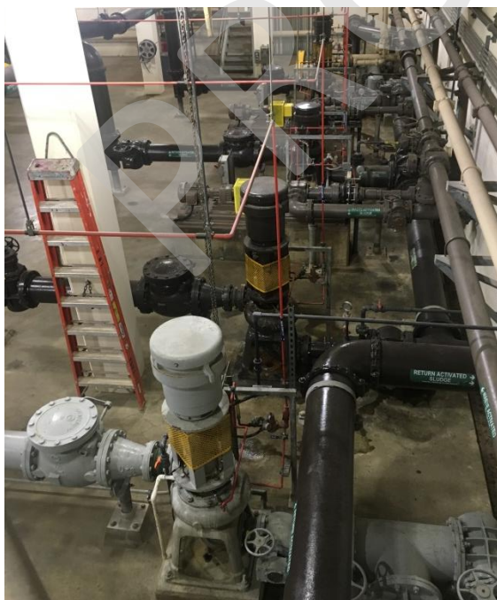
RAS and WAS pumps
