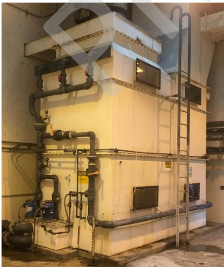
Headworks odor control scrubber
