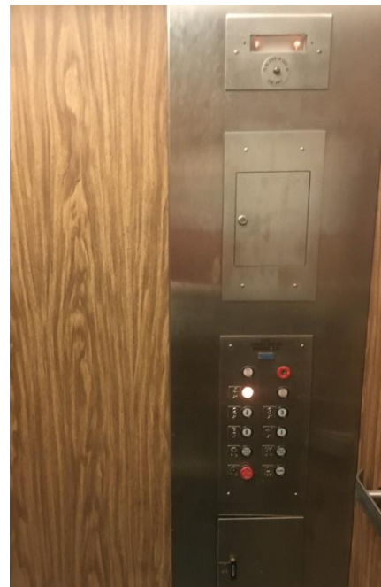
Elevator Control Panel
