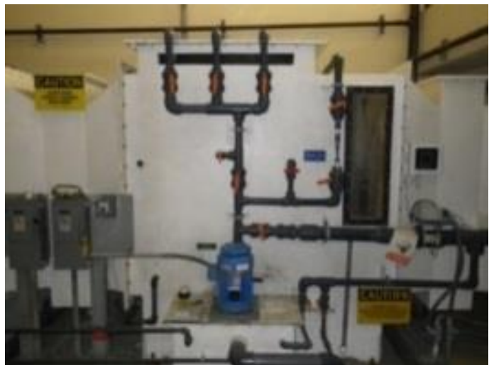
Solids Handling Building odor control scrubber
