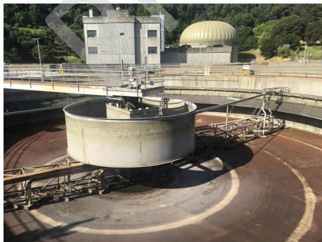
Secondary clarifier internal equipment
