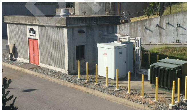
Switchgear building and transformer
