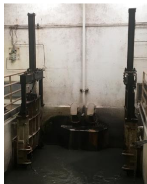
San Rafael and Ross Valley influent gates
