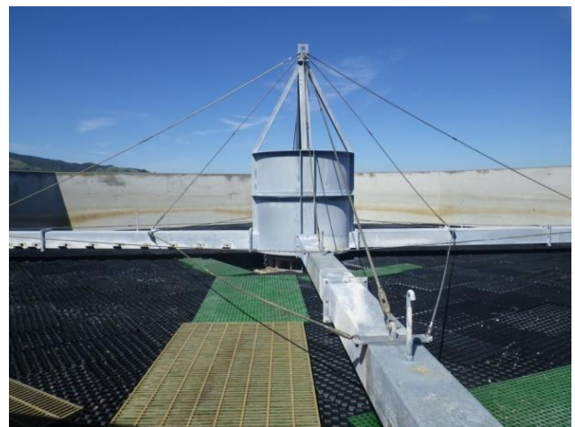
New rotary distributor, Biotower No. 2
