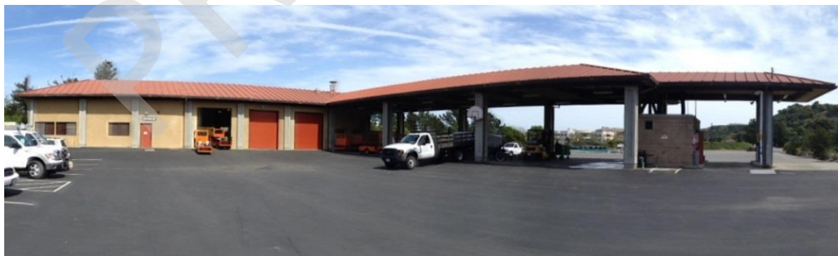
Maintenance Building with standing seam metal roofs.
