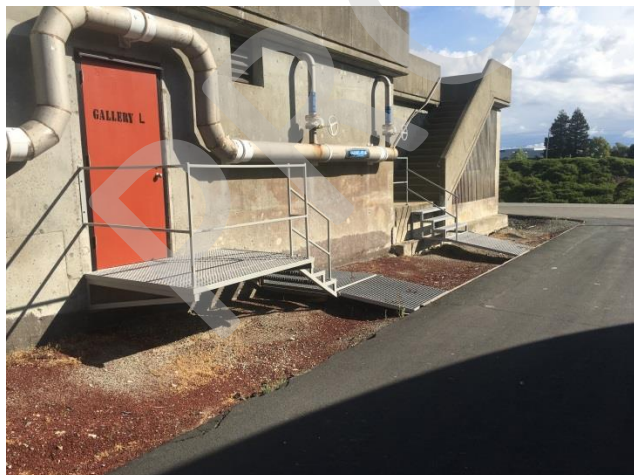
Stair modifications to account for settlement
