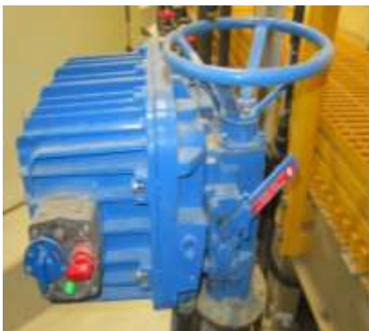
Original Motorized Valve Operator
