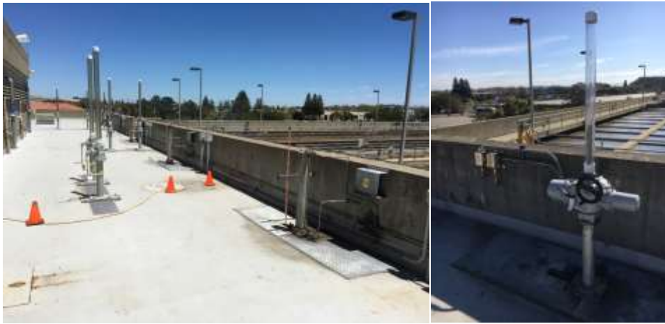
Old hydraulically-operated primary clarifier gate actuator systems (left) and new electric actuator(right)
