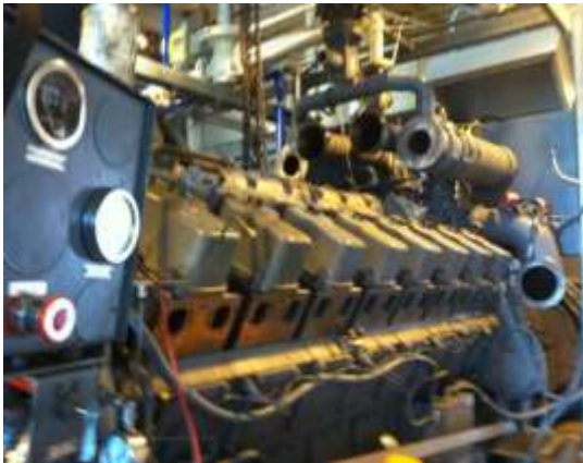
Cogenerator Equipment Removal
