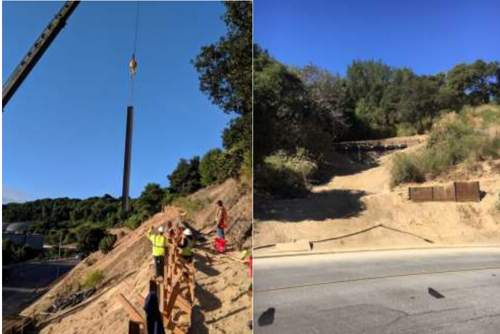
Retaining wall construction
