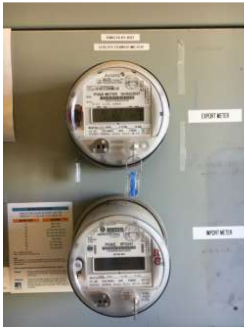
New power export meter (top)
