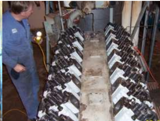
Inspecting Recently Installed Refurbished Cylinder Heads
