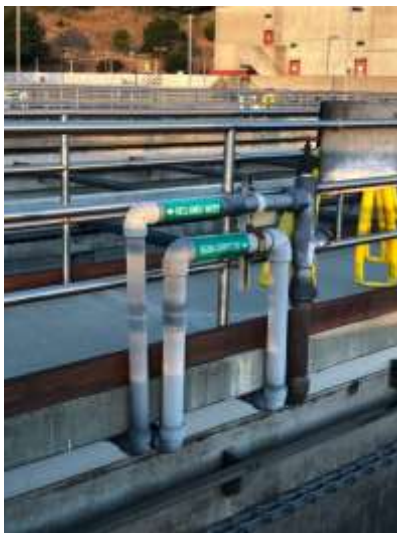
Original Reclaimed Water Piping
