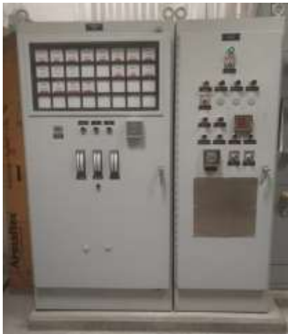
Existing Control Panel
