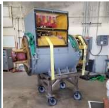
Generator Prepared for Offsite Repairs
