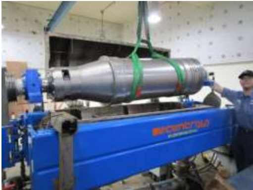
Centrifuge No. 3 Bowl Assembly Installation
