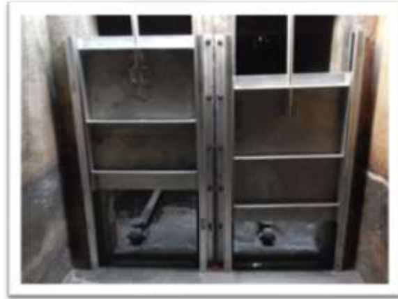
New Isolation Gates
