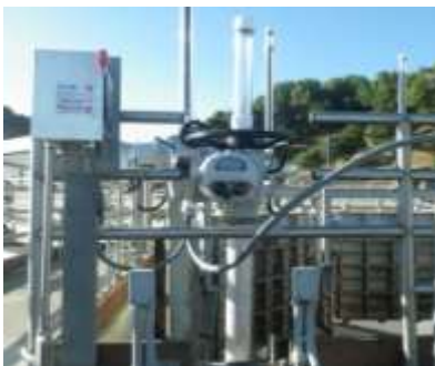
New Motor Operated Valve
