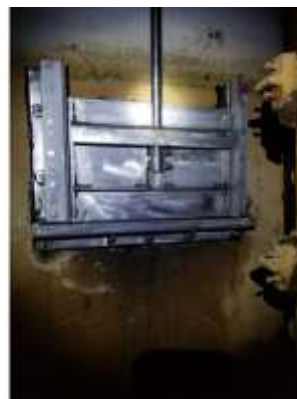
New Stainless Steel Isolation Gate
