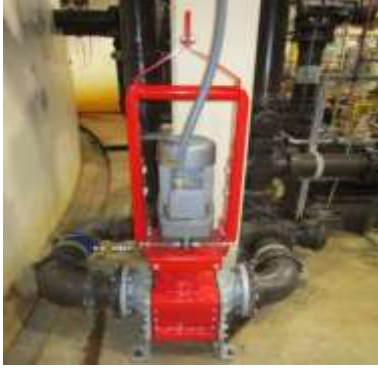
Sludge Grinder Cartridge and Piping
