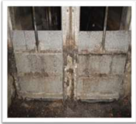
Originally Installed Isolation Gates
