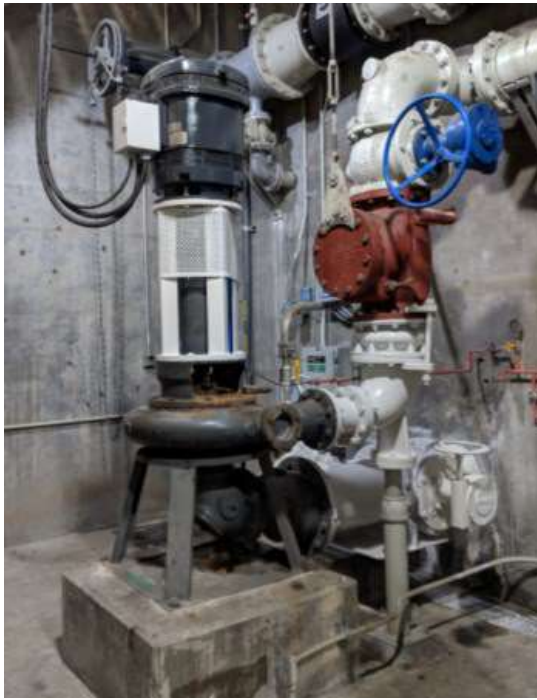
Direct-coupled pump with enclosed rotating equipment
