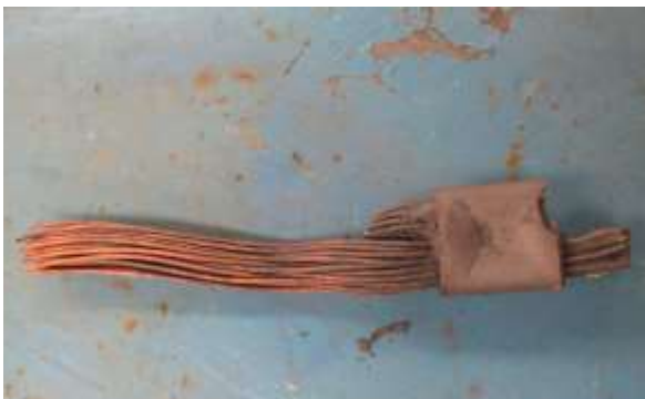
Copper Cable, Spot of Failure
