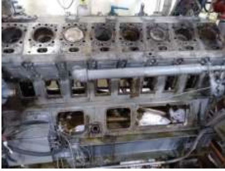
Cogenerator Apart after Failure
