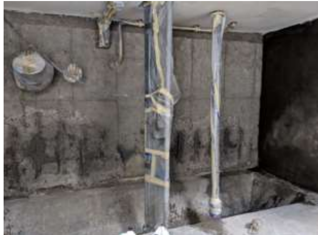
Spalled concrete in the hypochlorite drain vault
