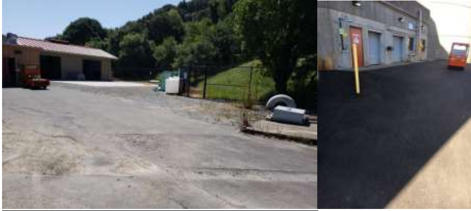
Deteriorated and newly placed pavement areas around the treatment plant
