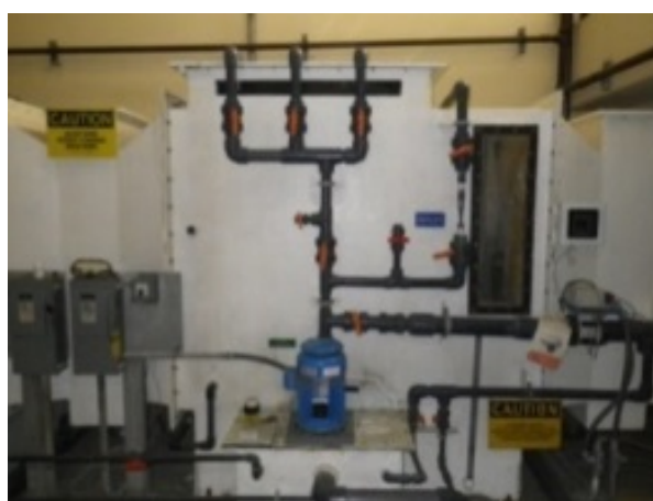
Solids Handling Building odor control scrubber
