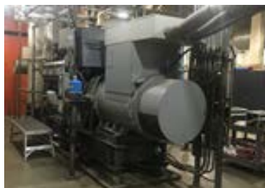
Existing cogeneration system
