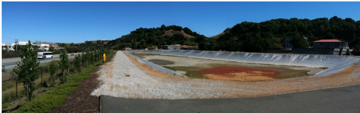
Effluent Storage Pond
