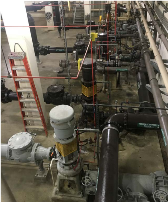
RAS and WAS pumps
