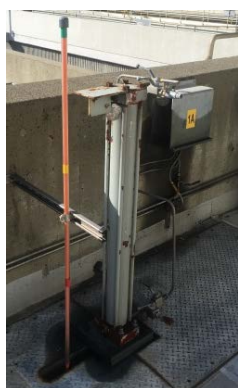
Hydraulic gate actuator
