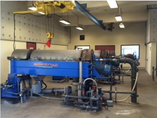
Existing Centrifuges
