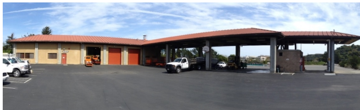
Maintenance Building with standing seam metal roofs
