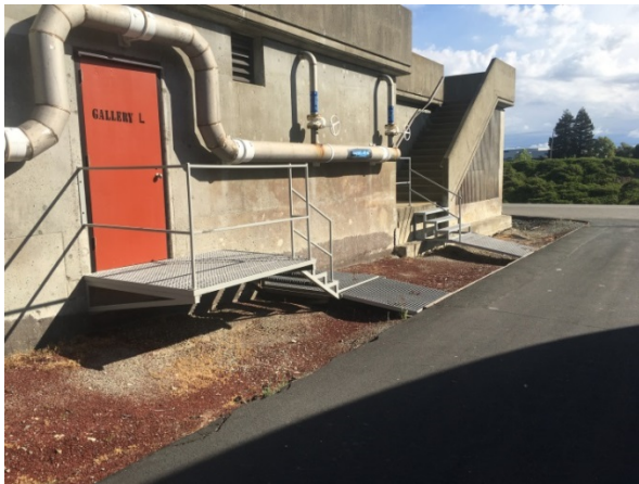
Stair modifications to account for settlement
