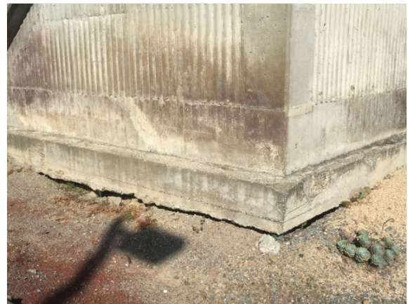
Exposed bottom of process tank
