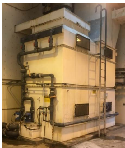
Headworks odor control scrubber
