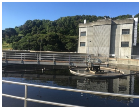
Secondary clarifier in operation
