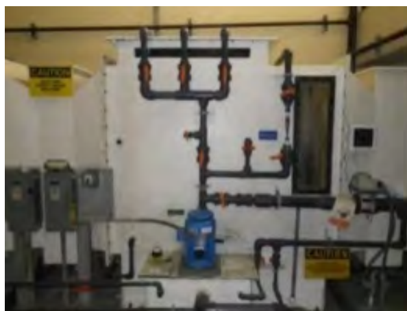
Solids Handling Building odor control scrubber
