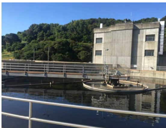
Secondary clarifier in operation
