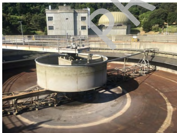
Secondary clarifier internal equipment
