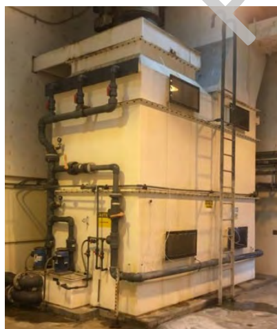
Headworks odor control scrubber
