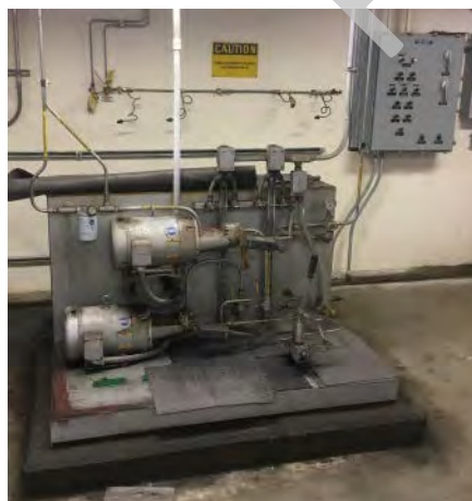
Hydraulic control system
