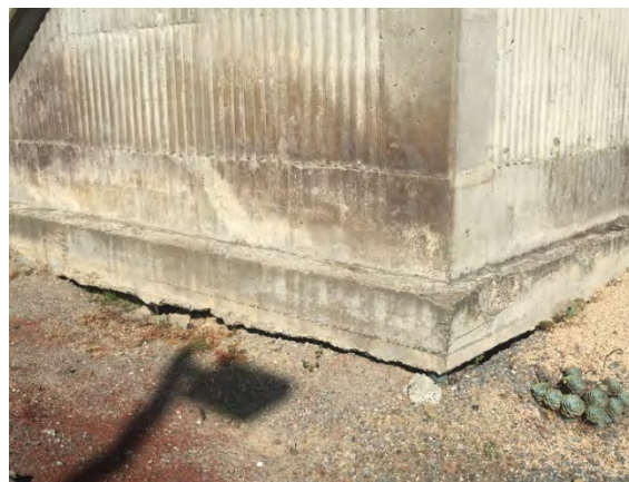
Exposed bottom of process tank
