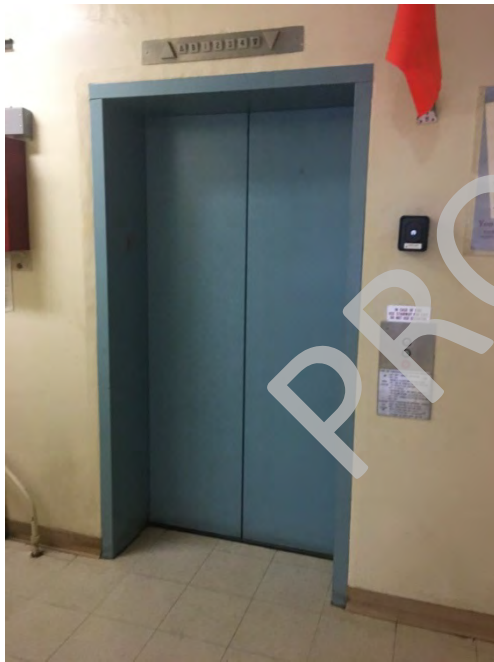
Solids Handling Building Elevator
