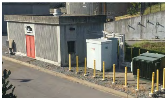
Switchgear building and transformer
