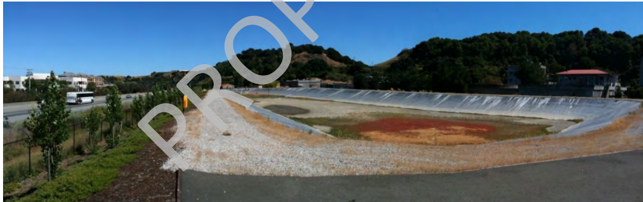
Effluent Storage Pond
