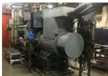
Existing cogeneration system
