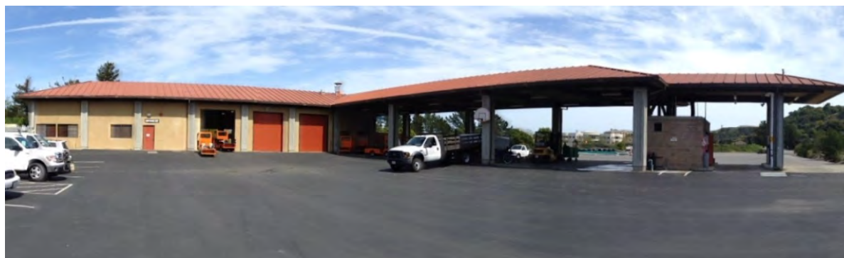
Maintenance Building with standing seam metal roofs
