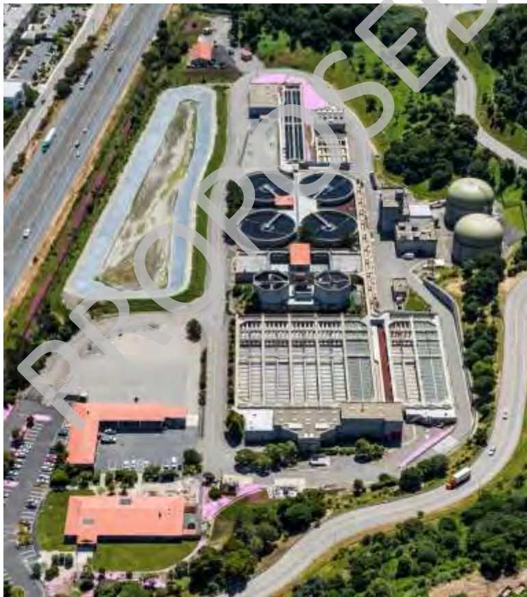
(Clockwise upper left to right): Effluent Storage Pond, Maintenance Annex (red roof behind the pond), Chlorination/Dechlorination Building, Chlorine Contact Tanks, Effluent Pump Station, Secondary Clarifiers, Organic Waste Receiving Facility, Solids Handling Building, Digesters and Digester Building, Aeration Tanks, Biotowers, Primary Clarifiers and Blending Channel, and Headworks. The two orange-roofed buildings in the lower left are the Maintenance Building (top) and the Administration Building (bottom).
