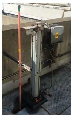
Hydraulic gate actuator
