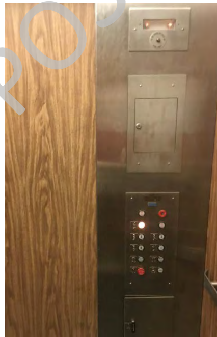
Elevator Control Panel
