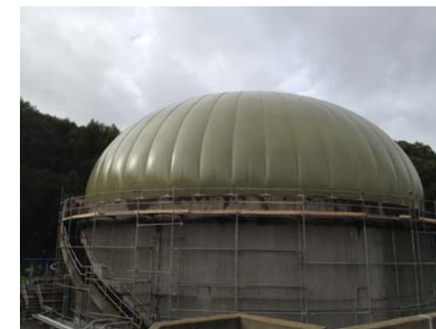
Replacement membrane cover inflated and ready for startup.
