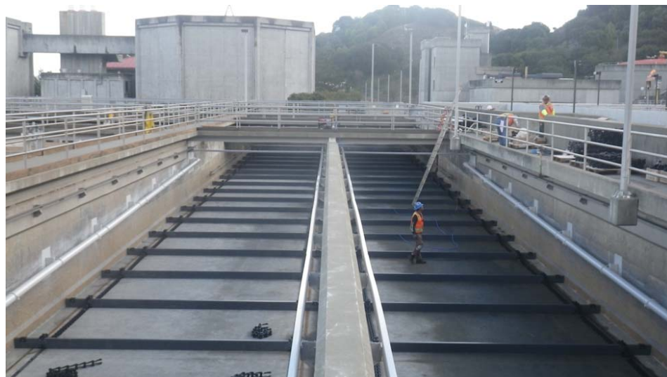
Primary Clarifier No. 1 with new sludge handlers being installed.
