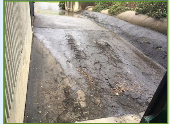
Failed pavement near the Ross Valley Interceptor.
