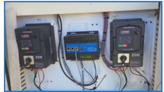
Peroxide pump controls.
