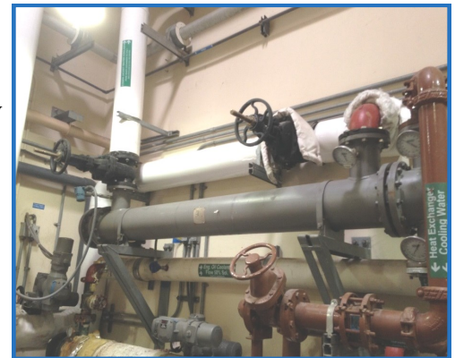
New waste heat exchanger.
