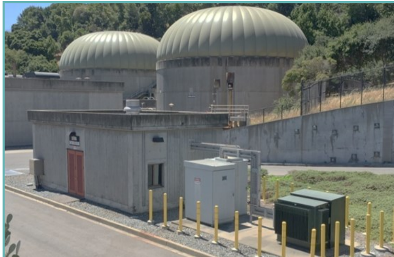
PG&E transformer (on right) and main plant switchgear (building on left); the Agency's two digesters in the background.
