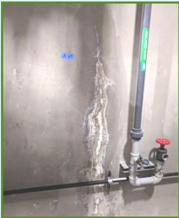
Gallery wall cracking.
